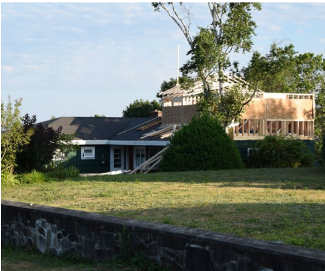
Residential construction in Lunenburg.
