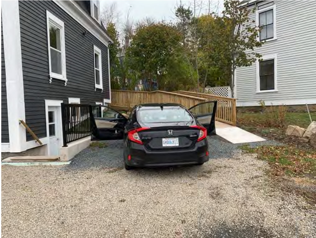
Figure 6 – Photo of the new off-street parking space
