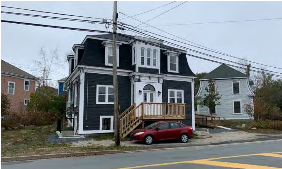
Figure 2 – Photo of the front façade.
