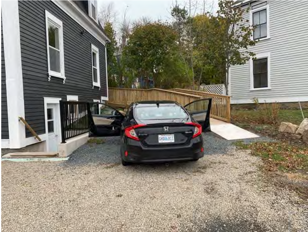
Figure 6 – Photo of the new off-street parking space
