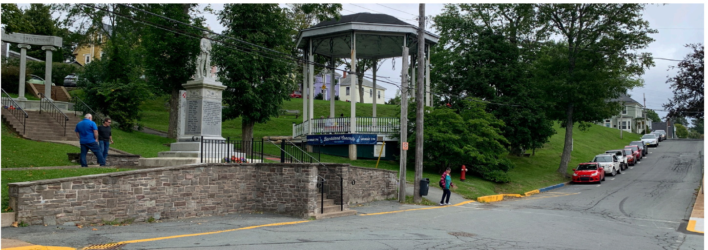
Image: Photo taken during the Design Team's initial site visit. View from Cumberland St.
