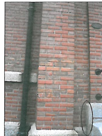
4. PILASTER FAILING.
