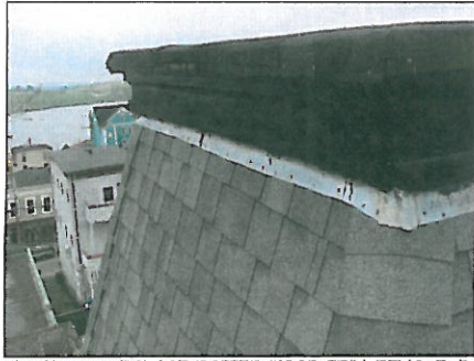
REPAIR OR REPLACE ROTTED WOOD TRIM, REMOVE NAILS ON LEAD & REPLACE WITH STAINLESS OR HOT DIPPED GALVANIZED.
