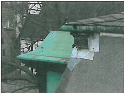
RECONDITION WOODWORK (L&S) INSPECT COPPER 58.
