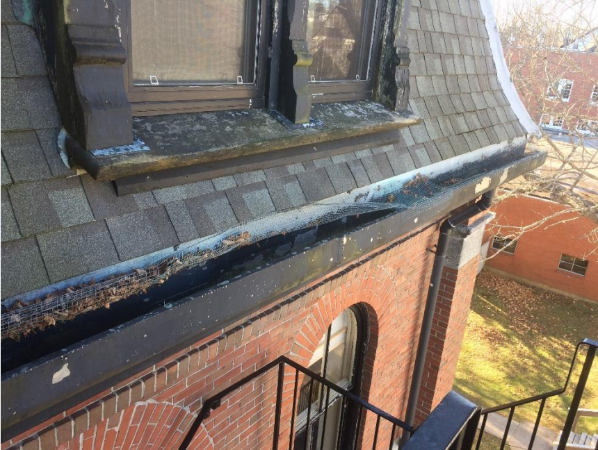
Photo 37 – Bent steel mesh above gutters
