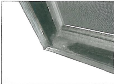
DAMAGED SILL, COURT ROOM WINDOW REPAIR LEAKS - INSPECT, REPAIR & CAULK 50.
