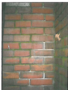
MOSS & BAD REPAIRS. 35. CLEAN AND REPOINT
