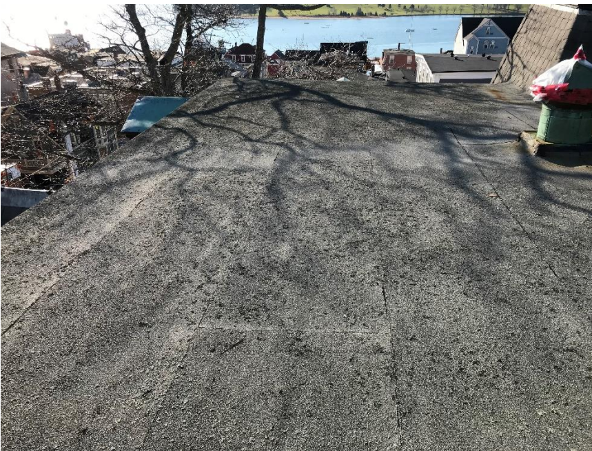
Photo 20 – Moss growth on roof membrane
