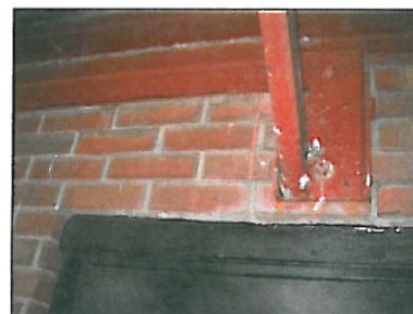
25. NO LINTEL AT NEW DOOR - CUT OUT BRICK AND INSTALL GALVANIZED LINTEL. SIZED TO SUIT
