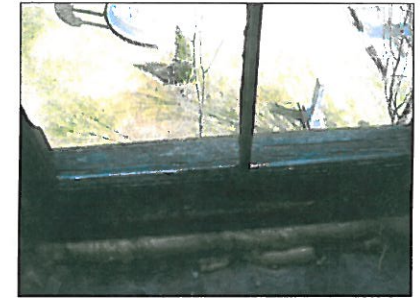
OLD SILL, REPAIR BEFORE CLADDING 49.
