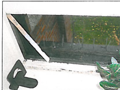
BATHROOM WINDOW, SPIKES IN SILL, REMOVE & REPLACE WITH SPECIFIED BIRD REPELLANT SYSTEM 51.
