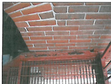
24. STRINGER AT LANDING - CORROSION. BLAST AND REPAINT
