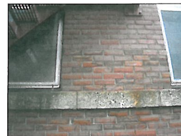
30. RUST ON STONE BAND COURSE - CLEAN POINT ALL JOINTS ON STONE TRIM - V4H
