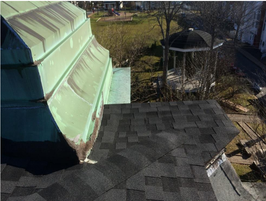
Photo 18 – Water-damaged shingles (2 of 2)
