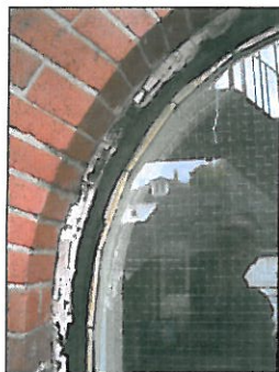
23. DETERIORATED TRIM, WIRED GLASS WINDOW - REPLACE/RECONDITON
