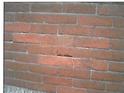
DAMAGED ORIGINAL BRICK WITH SMALL JOINTS. THIS IS DESIRED JOINTING FOR NEW BRICKWORK 44a.
