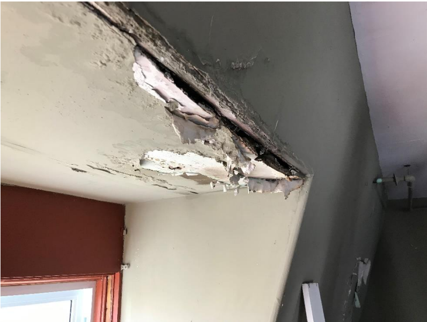
Photo 38 – Interior water damage, typical around dormers
