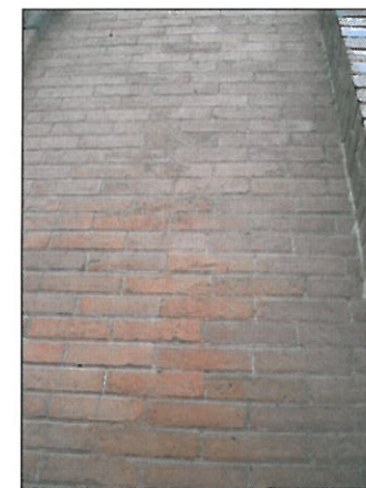
ABRADED ORIGINAL BRICK - INSPECT 44b. POSSIBLY TREAT (T+M)
