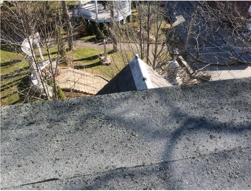
Photo 23 – Dormer with metal ridge cap
