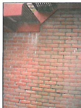
28. MOSS BUILD UP UNDER STAIRS. CLEAN / INSPECT. POINT AS REQ'D
