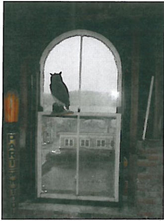
ATTIC - WINDOW TOP SASH DROPPED. (RC) 46.
