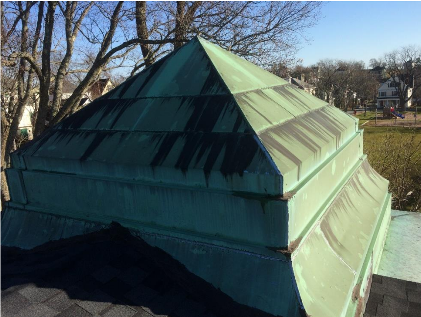
Photo 26 – Cupola with copper cover
