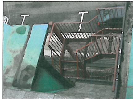
DORMER & FIRE EXIT INSPECT COPPER AS PER ALL COPPER, BLAST AND REPAINT STAIRS WITH SPECIFIED PAINT SYSTEM. 59.
