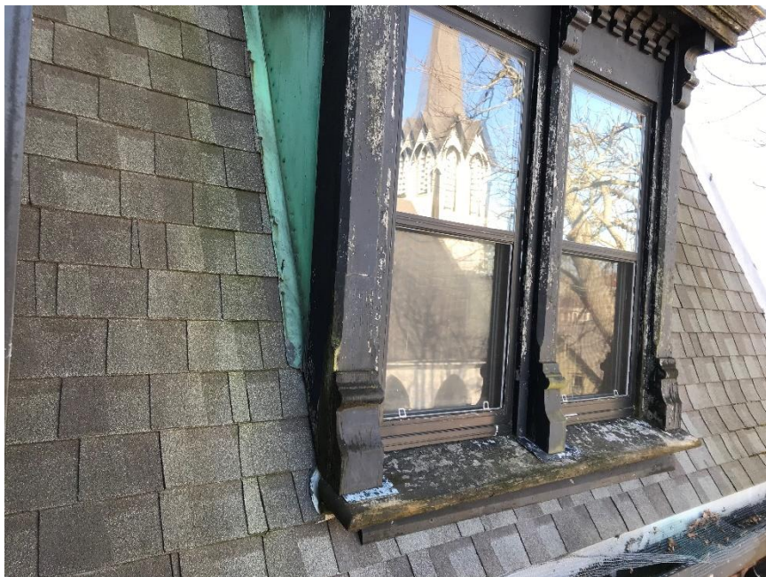
Photo 30 – Dormer with bent copper panel
