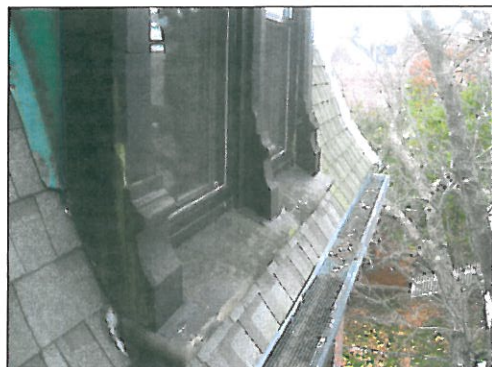
DOMER - WEATHERING, NEEDS REPAIR RECONDITION WOODWORK
