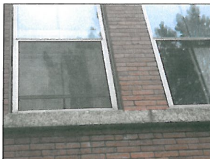
OPEN JOINTS - POINT ALL V+H JOINTS IN GRANITE (TYPICAL) 40.
