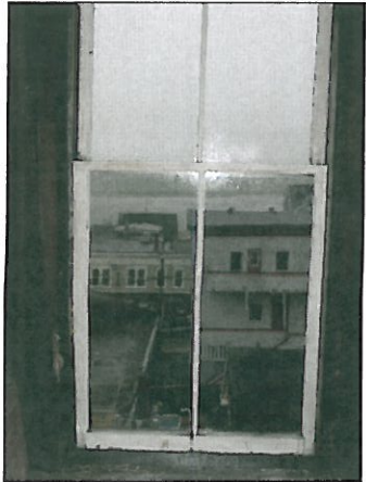
ATTIC WINDOW MISALIGNED. (RC) 45.
