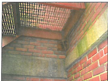
CORROSION TO FRAMES AND SUPPORTS. 31. BLAST PRIME AND PAINT, AS PER SPEC.
