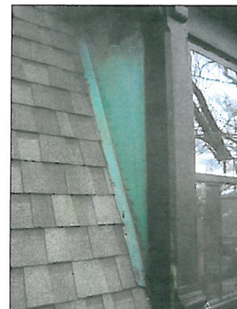
COPPER ON SIDE OF DOMERS, WRONG NAILS 19. REPAIR / RECONDITION
