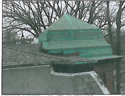
INSPECT COPPER - ADVISE ON REPAIRS UNDERTAKE AS APPROVED ON (T&M BASIS) REPLACE ALL NON COPPER NAILS WITH COPPER (L&S)
