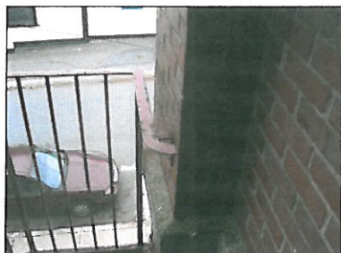
RUST ON RAILING - BLAST PRIME AND PAINT 32.
