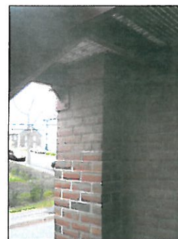
29. POORLY MATCHED REPAIR. CUT OUT AND REPOINT
