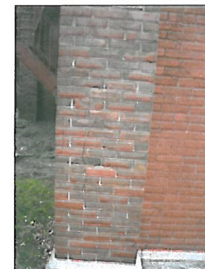
STRESS CRACK, SAME PILASTER 38. REBUILD
