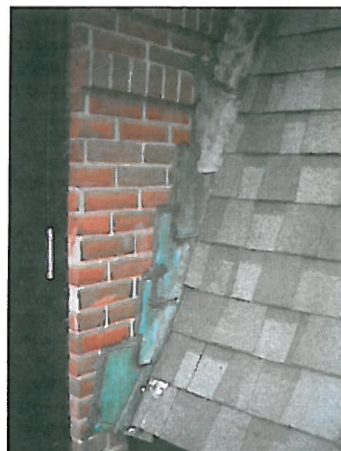
STEP FLASHING ROOF/TOWER LEAD & COPPER
