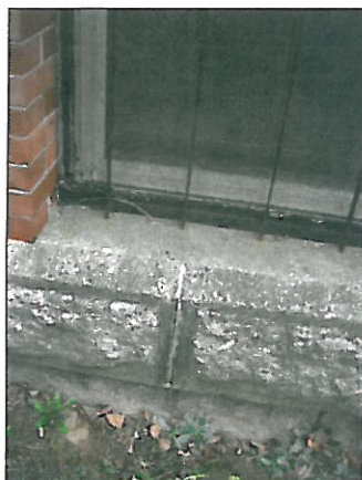
OPEN SILL JOINT GRANITE - POINT - TYPICAL 39.
