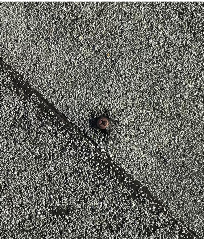
Photo 22 – Screw in roof membrane (2 of 2)
