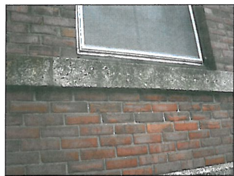
JOINT FAILURES - CRACKED BRICK 36.
