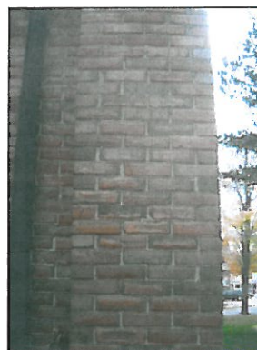
CRACKED BRICK PILASTER 37. REBUILD
