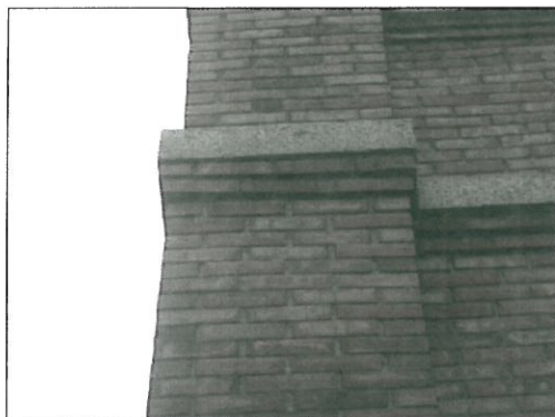
3. POOR REBUILT CORBEL ON PILASTER - REBUILD
