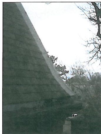
GUTTER, PAINT FLAKING - REPAINT
