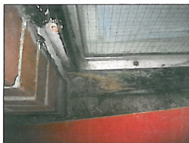
27. ROTTEN SILL - WIRED GLASS WINDOW. REPALCE / RECONDITION
