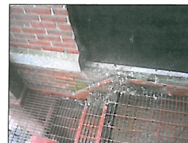
26. BIRD GUANO - REMOVE, BLAST STEEL AND REPAINT
