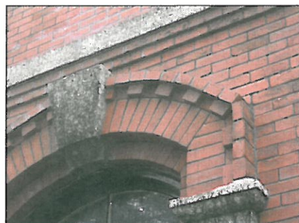
SOME MISSING BRICKS IN ARCHES - REPAIR ALL BRICK ARCHES TO BE 100% REPOINTED 42.
