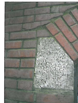
MOSS BUILD UP ON JOINTS - 34. CLEAN AND POINT WHERE REQ'D
