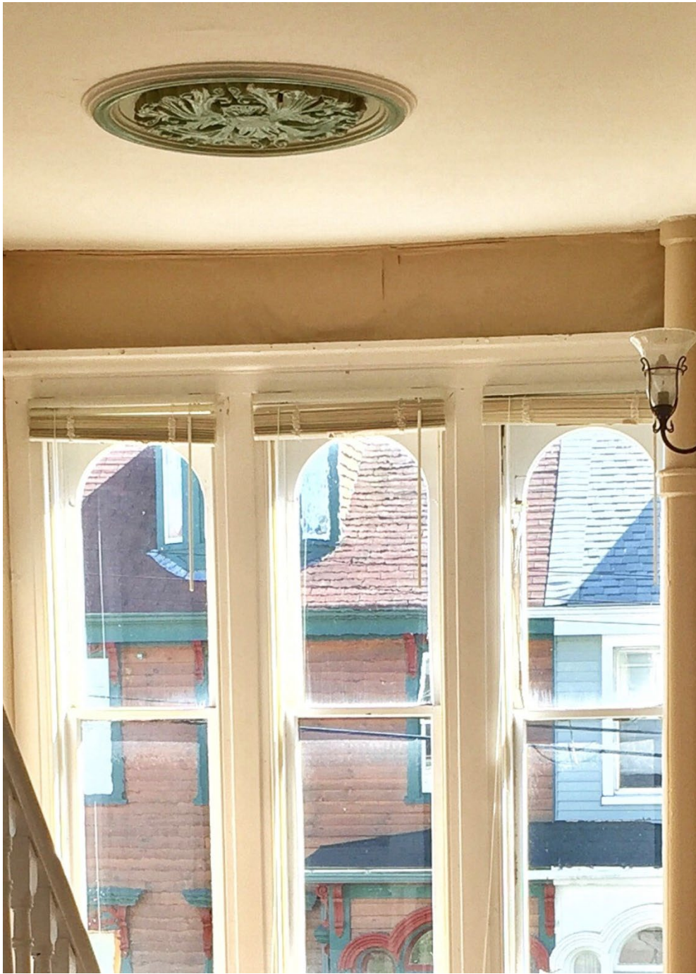
Figure 1: Photograph Supplied by Owner, dated by owner September 13, 2016
