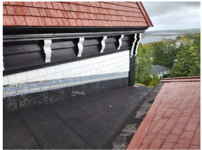
Existing – mod. bit. at sidewall of tower
