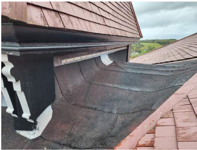
General – Existing saddle at backside of tower
