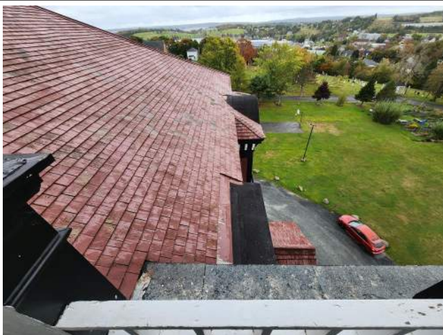
View from tower looking towards eye-brow dormer
