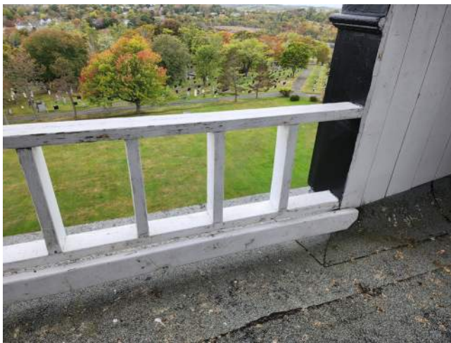
General – Existing Railing, Mod. Bit. at tower
