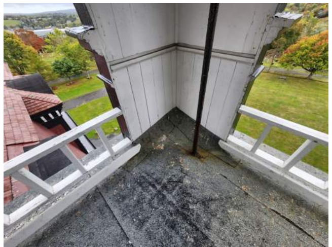
General – existing mod. bit., penetration at tower
