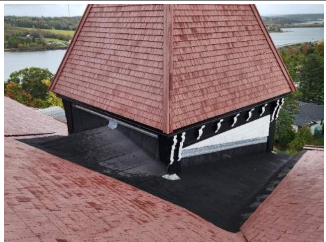
General – Mod. Bit. at Towers
