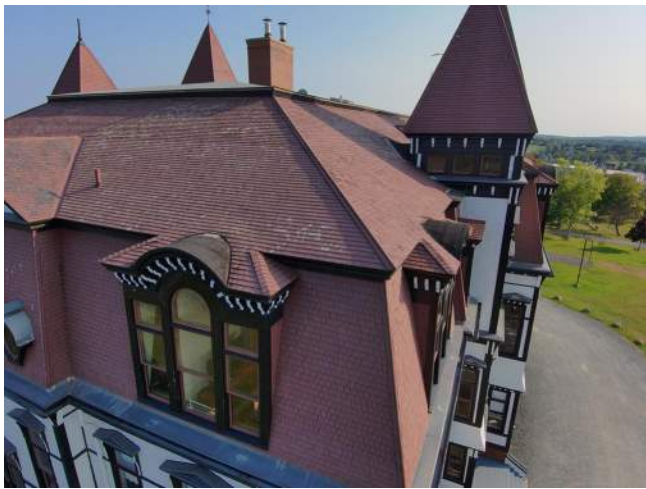
General – Sloped roof area and eye-brow dormer
