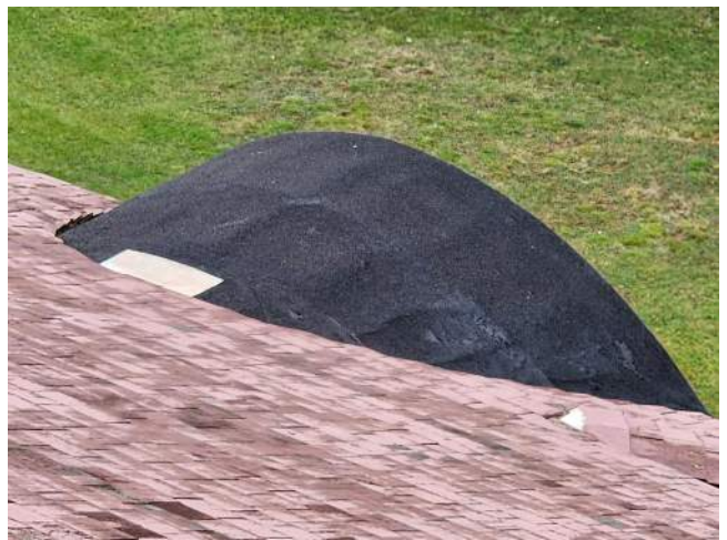
General – existing conditions – eyebrow dormer
