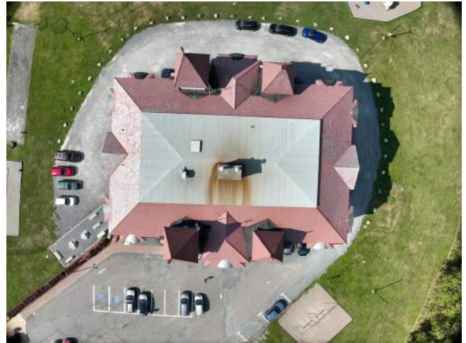
General Overhead – Mod. Bit.
