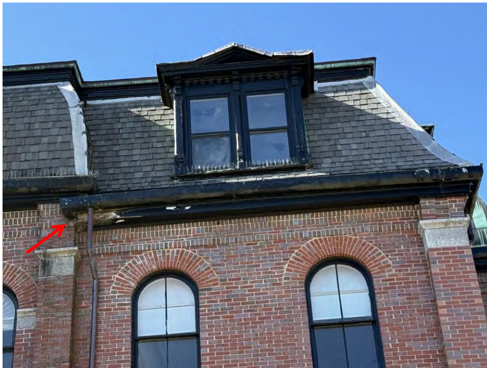
Photo 6: Overview of deteriorating wood trim at eavestrough
