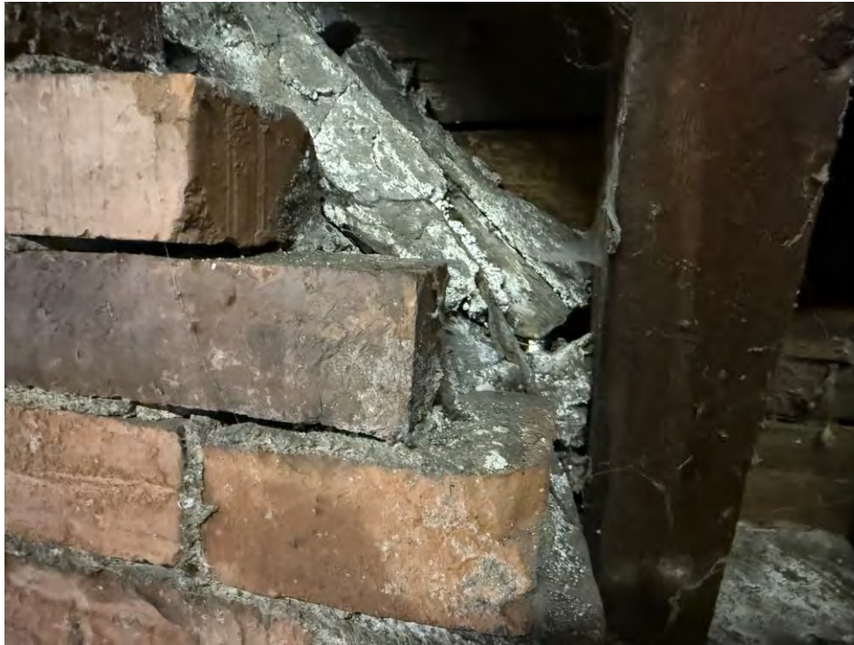
Photo 27: Daylight at window opening in attic/storage space
