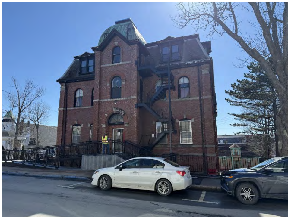
Photo 2: Overview of Town Hall north elevation (Townsend Street entrance)
