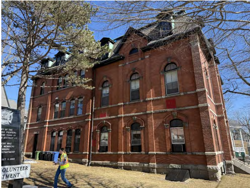
Photo 5: Overview of Town Hall west elevation
