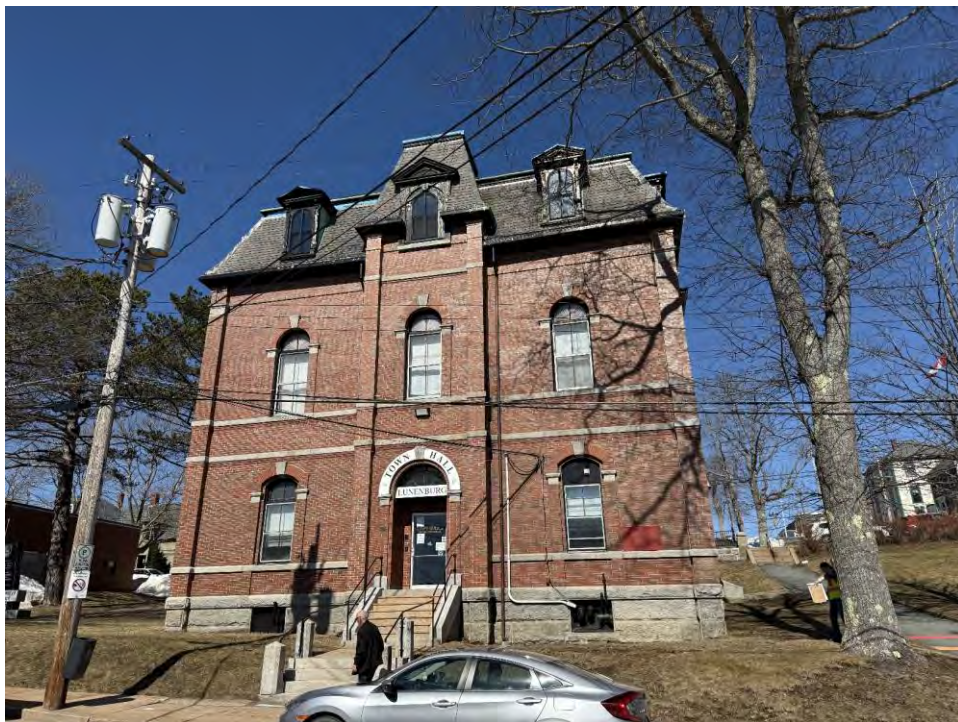
Photo 4: Overview of Town Hall south elevation (Cumberland Street Entrance)
