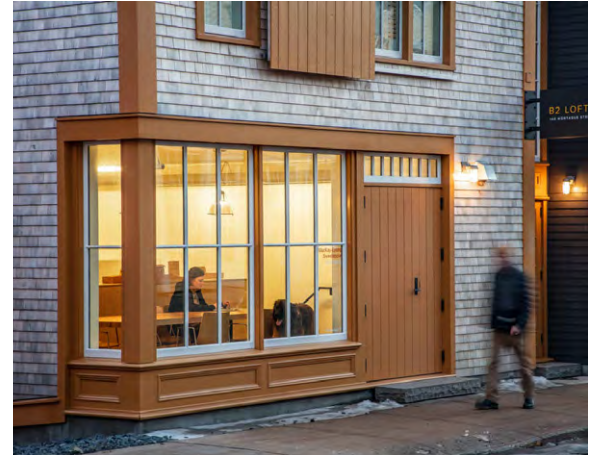
CORNER AT B2 LOFTS
