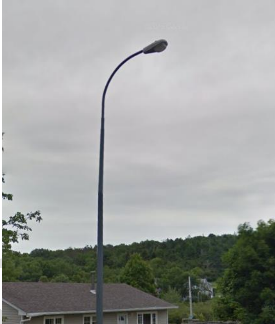
Figure 5: HPS Lighting Fixture Installed on Centennial Avenue
