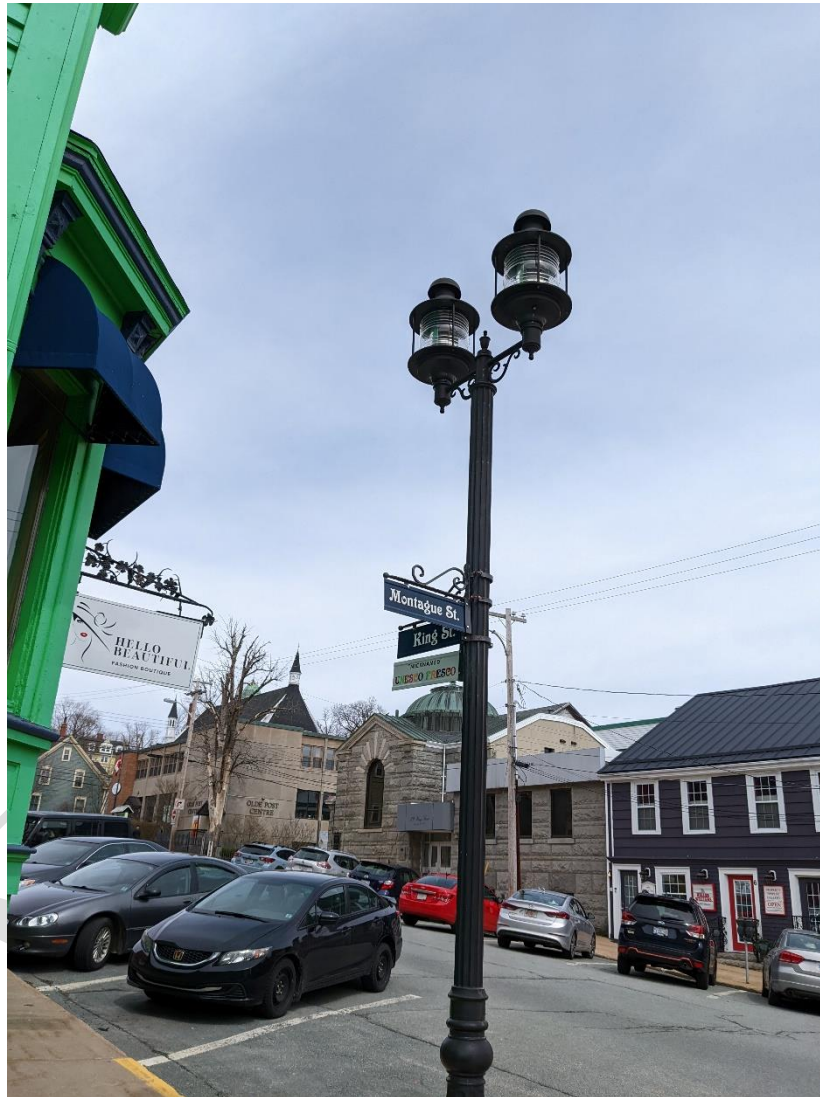
Figure 8: Historic Lighting Fixture Style 3 Dual Fixture Installed on a Custom Pole
