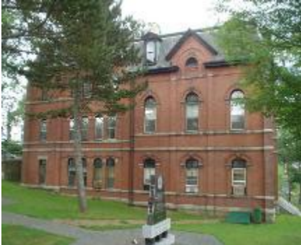
Town Hall, west elevation
