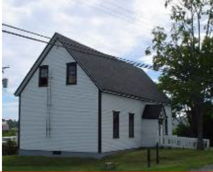
Front and North West Facades
