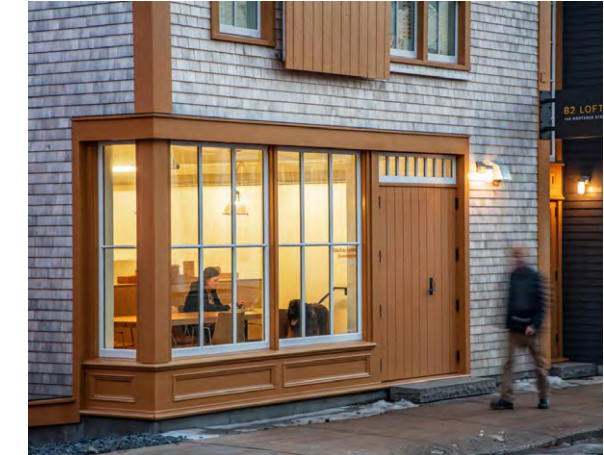
CORNER AT B2 LOFTS
