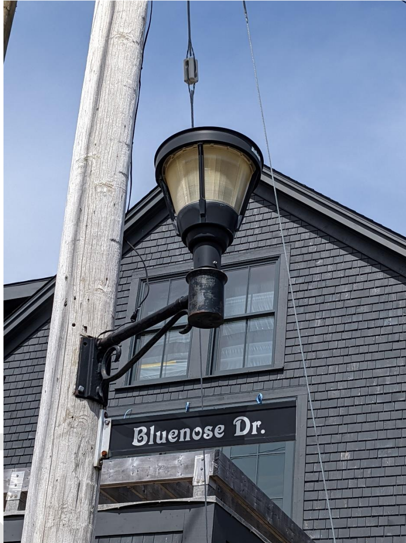
Figure 6: Historic Lighting Fixture Style 1 Installed on a Utility Pole
