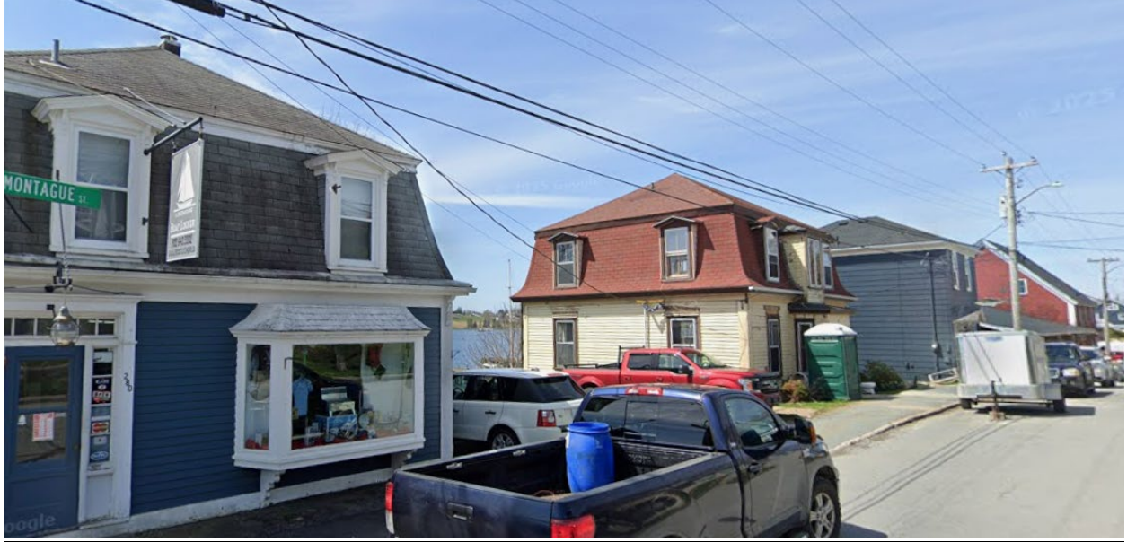
Figure 2 Montague Streetscape, Mansard Roof Residential within Marine Form Zone
