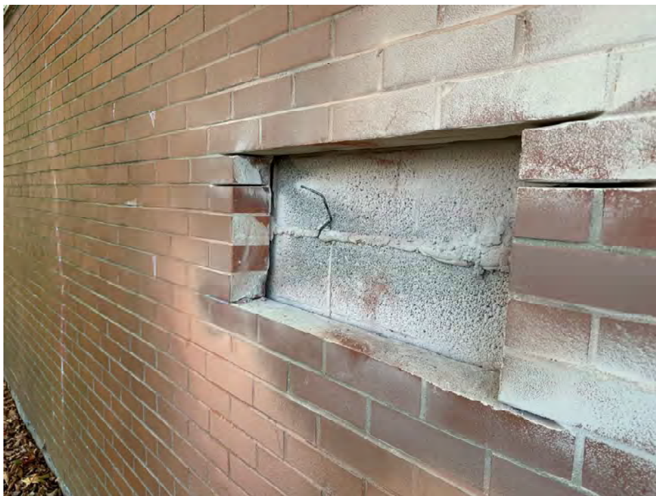
Photo 24: Exploratory brick opening on north elevation
