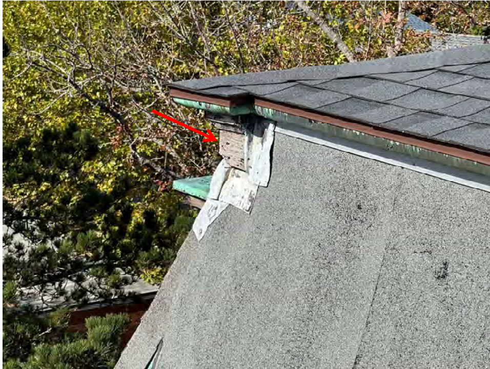
Photo 15: Modified bitumen roofing termination below asphalt shingle roofing
