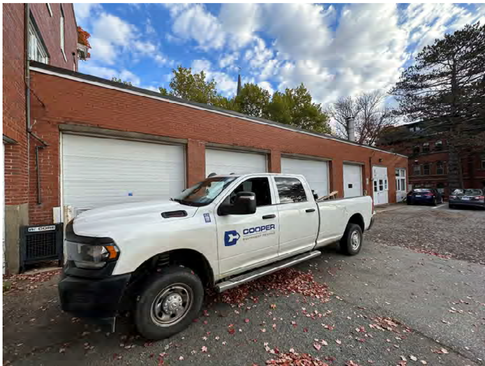
Photo 2: Overview of Electric Light Shop south elevation
