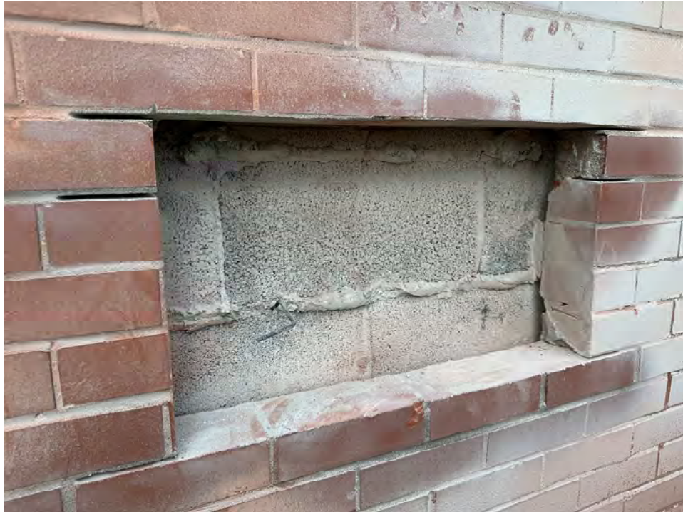
Photo 23: Exploratory brick opening on east elevation
