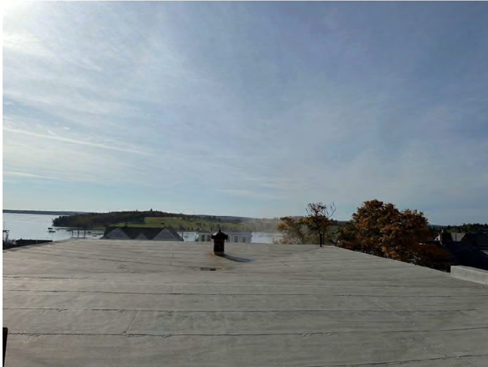
Photo 14: Overview of existing roofing membrane
