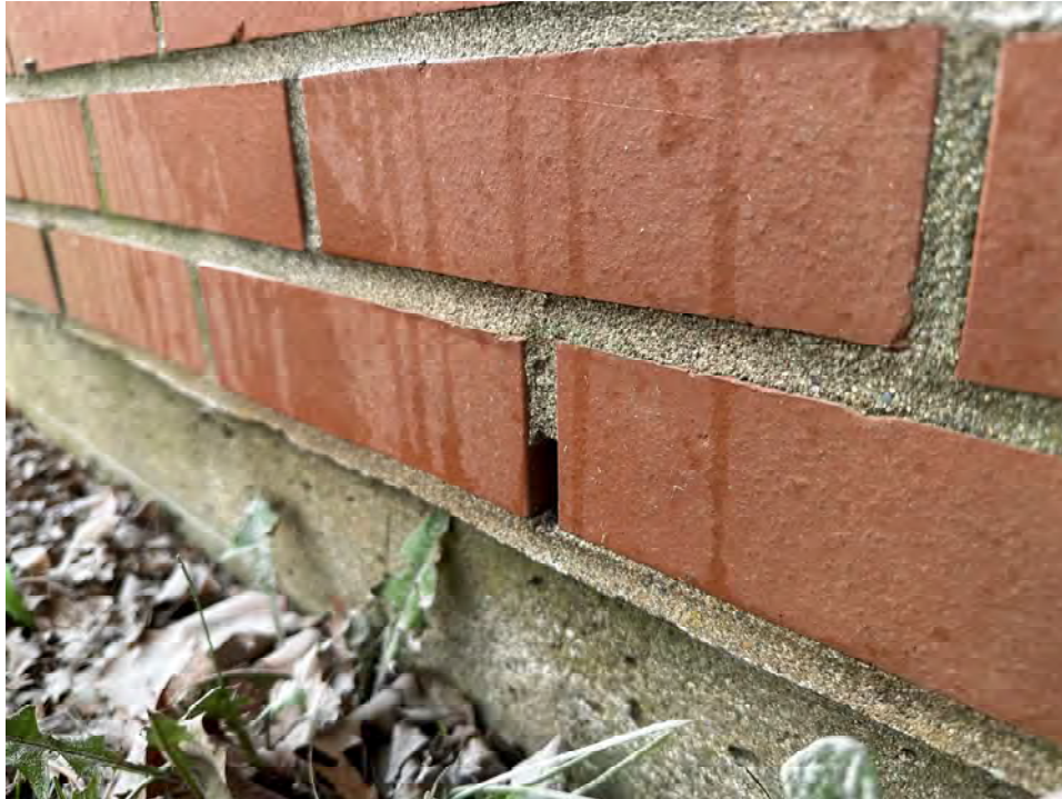
Photo 7: Close-up of weep hole at base of north elevation exterior brick
