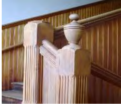
Interior staircase detail
