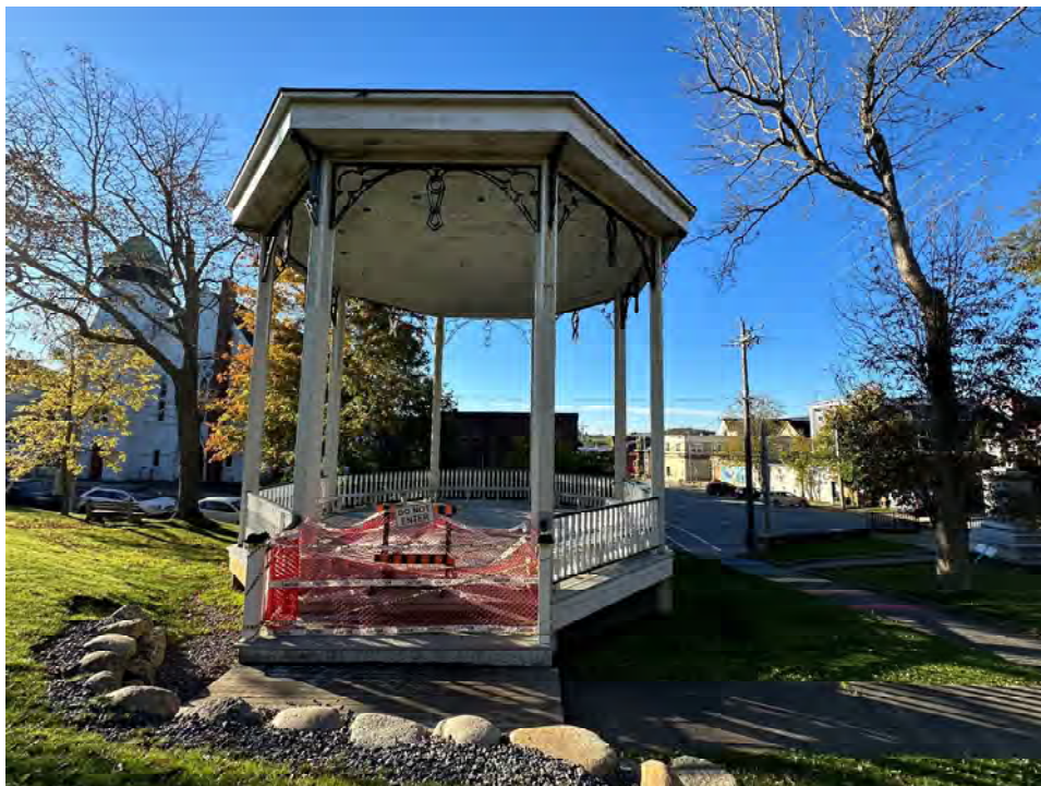
Photo 2: Overview of Bandstand north elevation (facing Cumberland St.)
