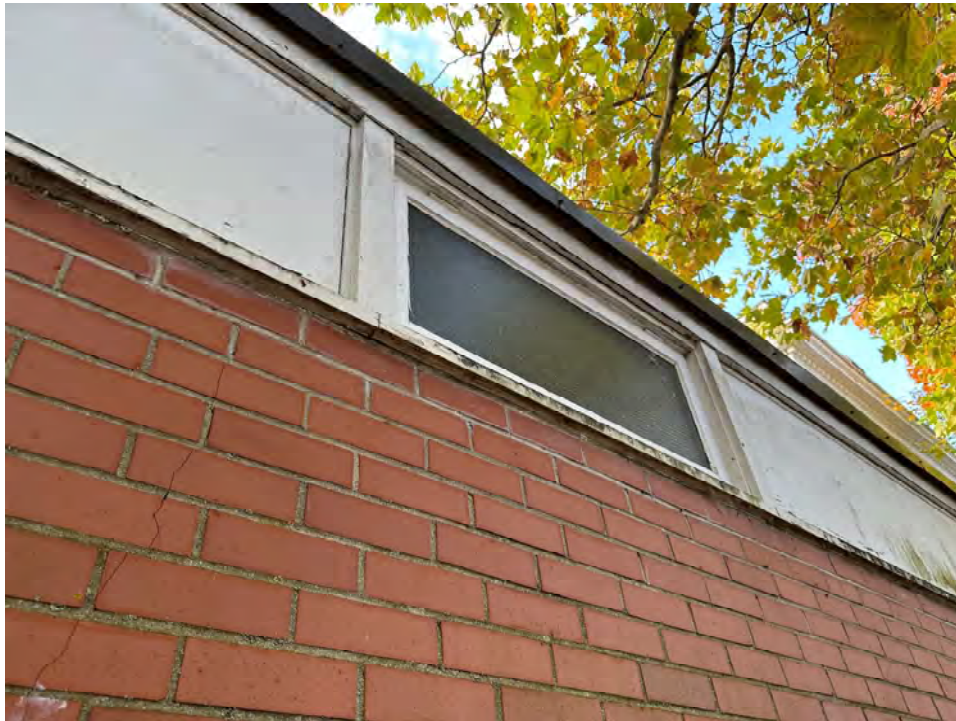
Photo 19: Wood-framed window and plywood coverings on north elevation wall
