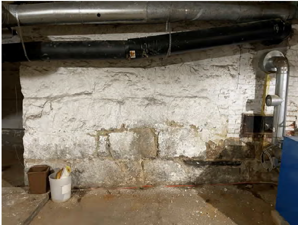
Photo 43: Stone foundation wall
