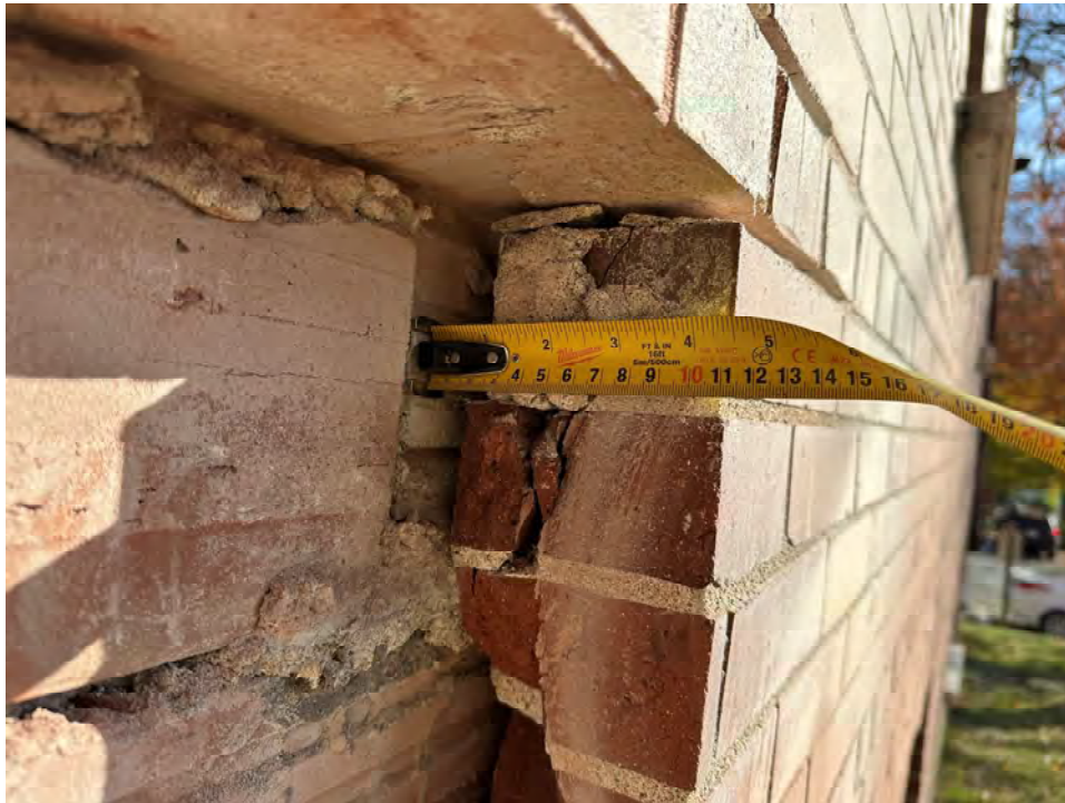
Photo 19: Exploratory brick opening on south elevation
