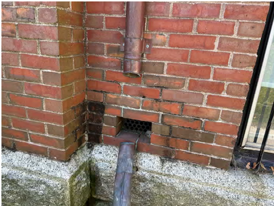
Photo 10: Copper downspout (note discontinuity)
