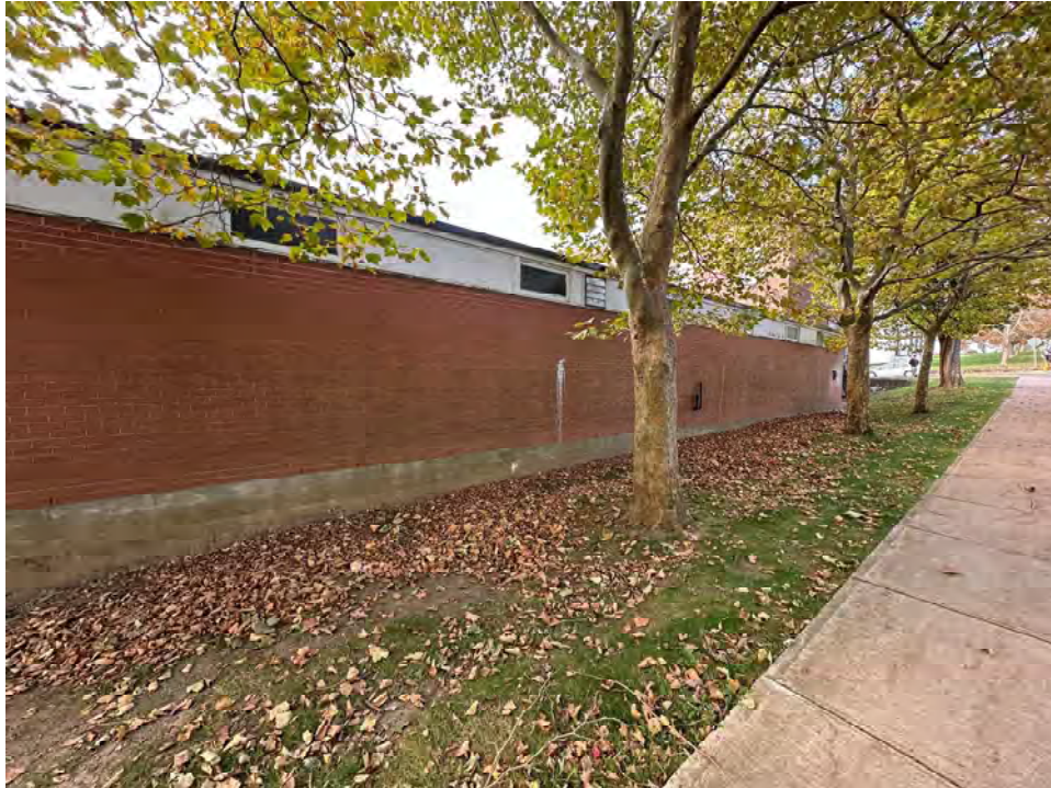
Photo 3: Overview of Electric Light Shop north elevation
