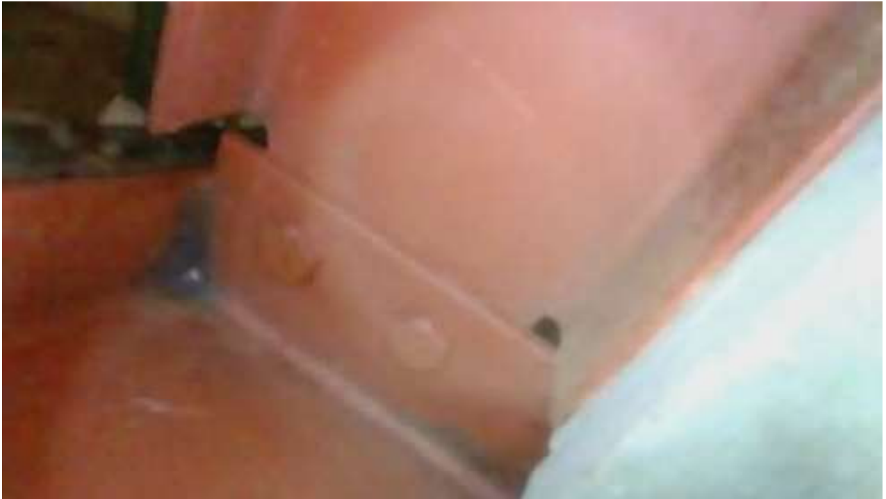
Photo 7: Borescope image of roof steel connection
