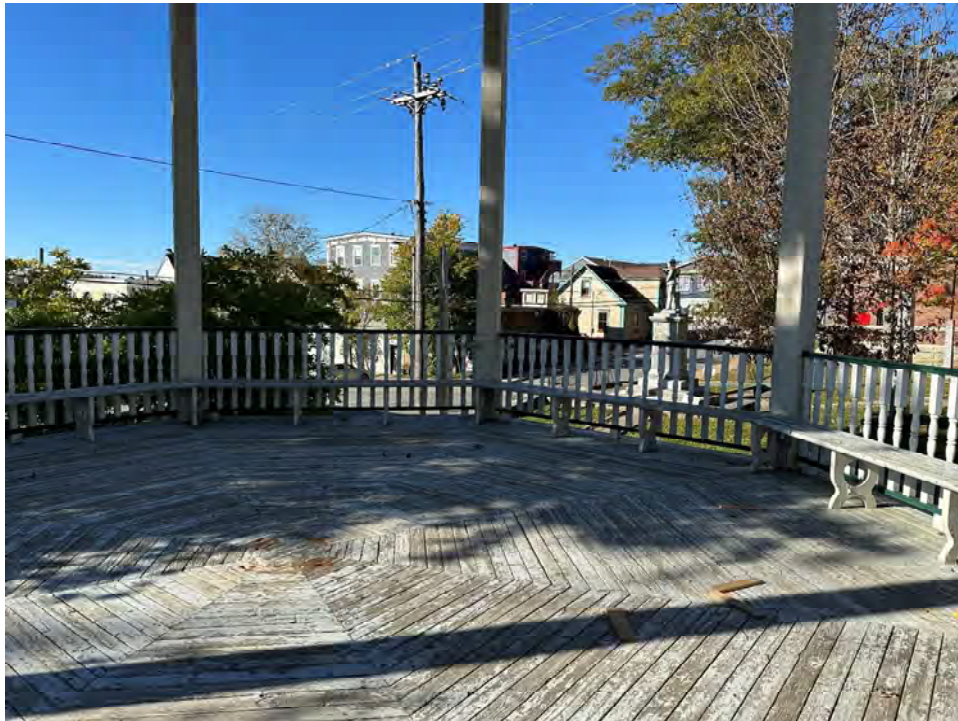
Photo 9: Overview of wood decking, benches and guardrails
