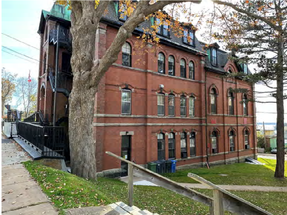
Photo 5: Overview of Town Hall west elevation
