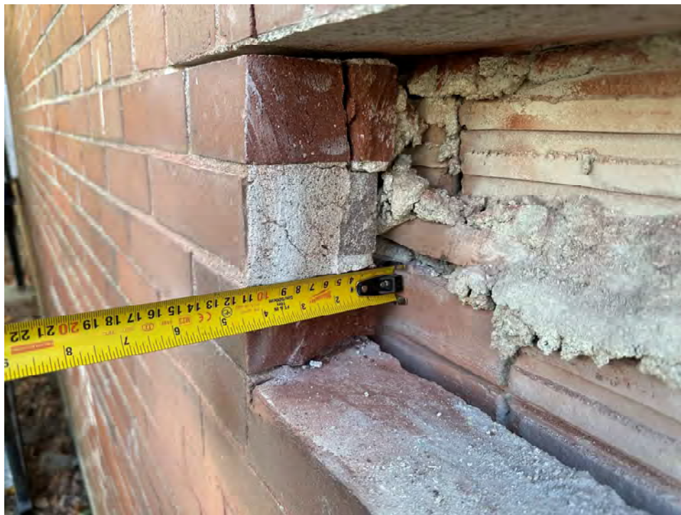
Photo 18: Exploratory brick opening on north elevation
