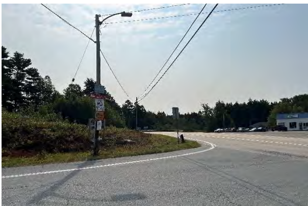
Photo 1: Route 332 Southbound Looking East
