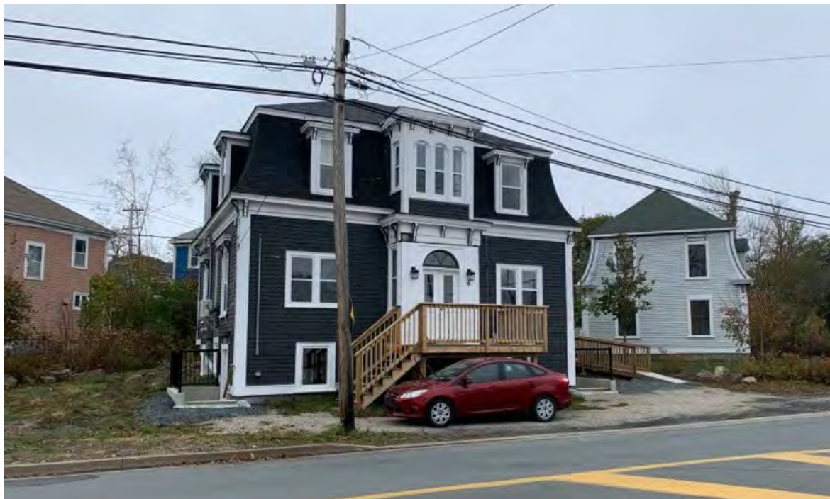
Figure 2 – Photo of the front façade.
