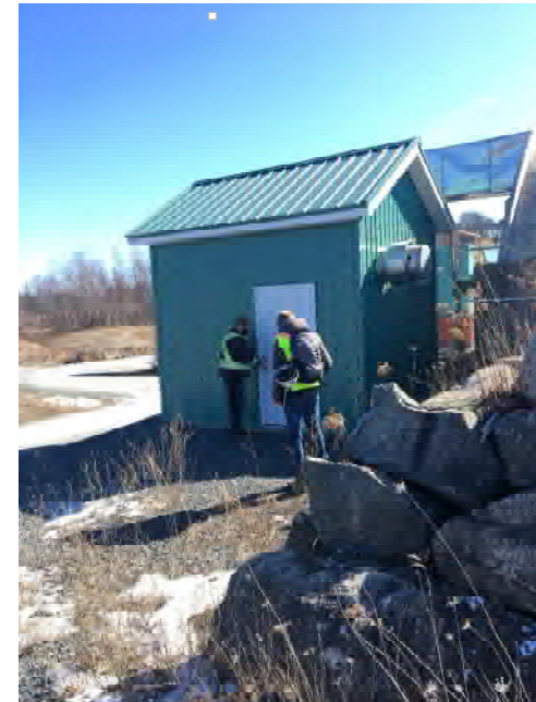
Biofilter Fan Building
