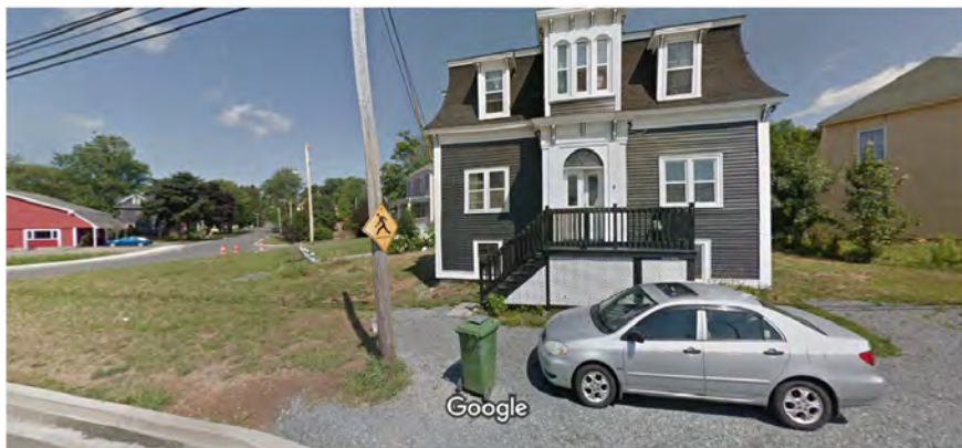
Figure 4: Photograph of home after exterior renovations in 2018 and installation of curbs and new municipal infrastructure.
