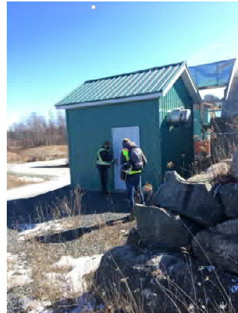
Biofilter Fan Building
