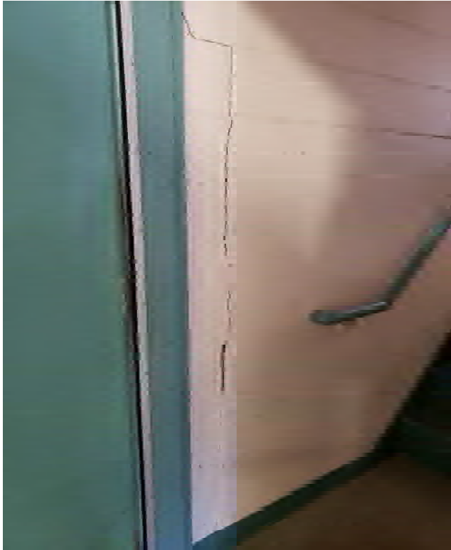
Crack in basement/foundation wall, near entrance to process area (south side of hallway).
