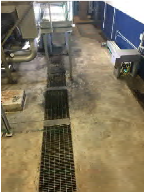
Floor slab in Process Room 112
