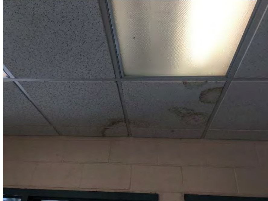
Acoustic tile in Office 109
