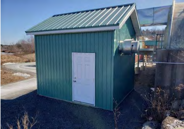
North elevation of the Biofilter Fan Building; note near-new condition
