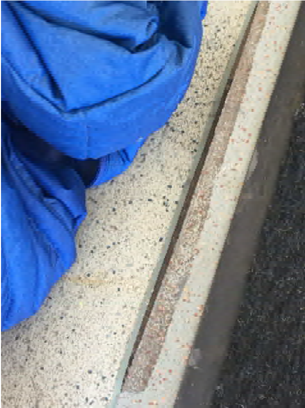
Vinyl Flooring in Entry 101
