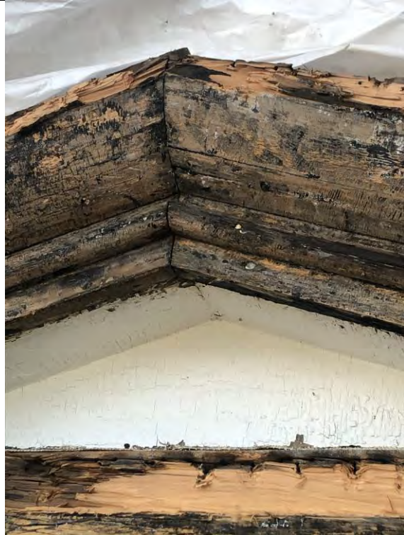
Figure 40 – Pediment. Rotten wood and missed parts.
