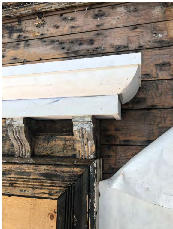
Figure 50 – Pediment bottom part repaired.
