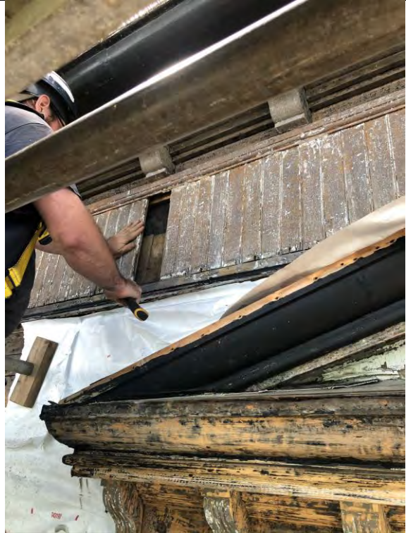
Figure 32 – Note removed planks to be repaired above pediment.
