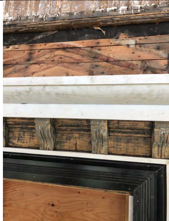
Figure 31 – Pediment to be disassembled and repaired. Rotten wood at corner.
