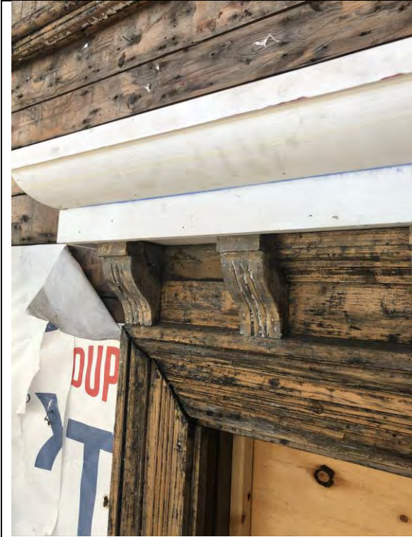
Figure 47 – Pediment partially repaired and primed.
