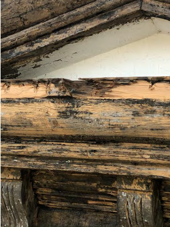
Figure 35 – Pediment to be disassembled, repaired, and reassembled. Broken wood detail.
