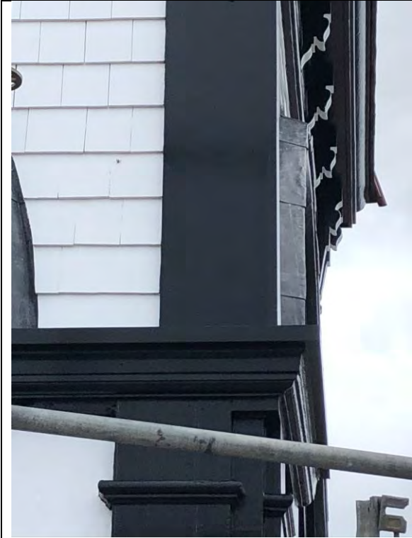
Figure 7 – Lead coated copper flashing on tower arched opening. Side view.
