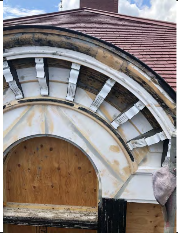
Figure 16- Wood work being repaired at the Palladian windows. Note dutchmen repairs.
