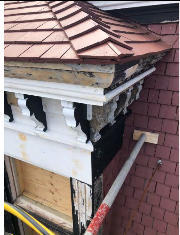
Figure 14- Wood work being repaired at the Palladian windows
