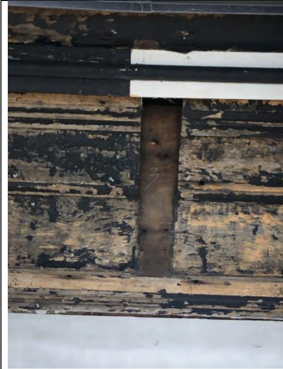
Figure 55 – Cornice with removed corbel being repaired.
