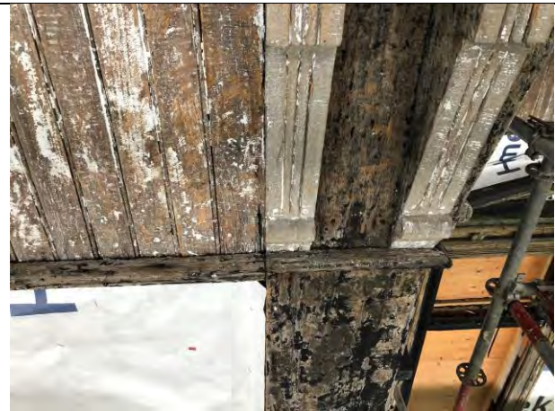
Figure 10– Siding on the 3 rd floor elevation- paint is removed. Wood is in good condition.
