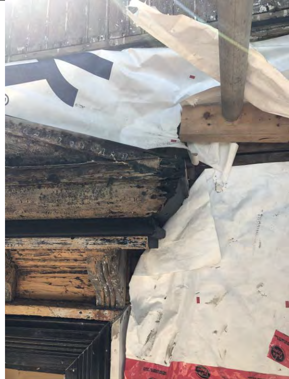
Figure 31 – Pediment to be disassembled and repaired. Rotten wood at corner.
