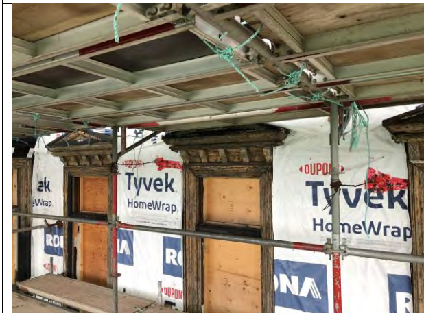
Figure 11 – Windows trims, sill and transom sills. Paint is removed and existing bare wood is exposed.
