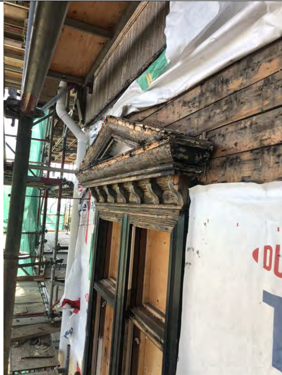
Figure 40 – Pediment. Rotten wood and missed parts.
