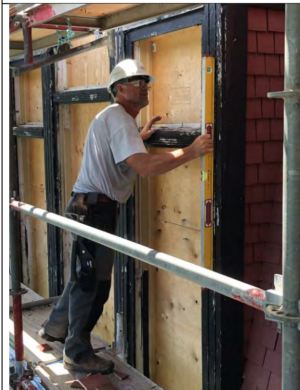
Figure 19 –Out of plumb of widows being verified.
