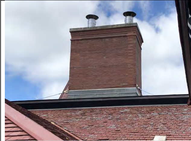
Figure 5 – Zoom in on the area of roof re-shingle to be completed.
