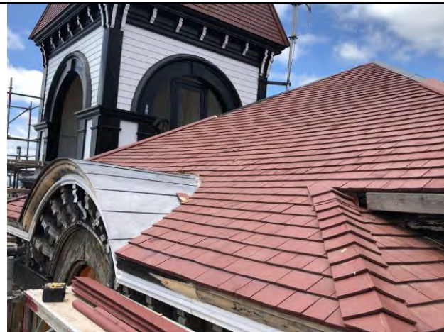
Figure 3 – Area of roof re-shingle almost complete
