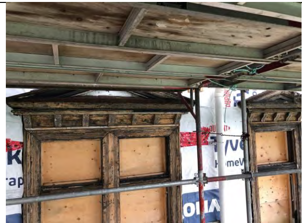
Figure 12 – Shingles on the elevation are removed and permeable membrane is being installed.
