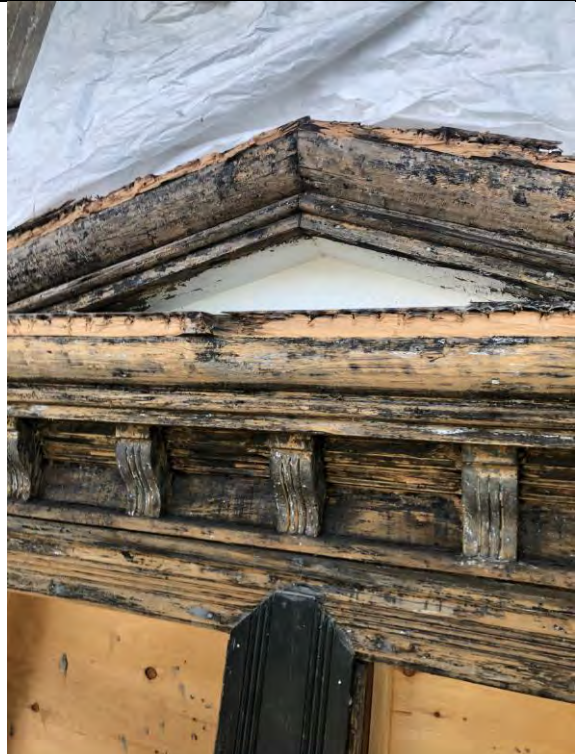
Figure 32 – Note removed planks to be repaired above pediment.
