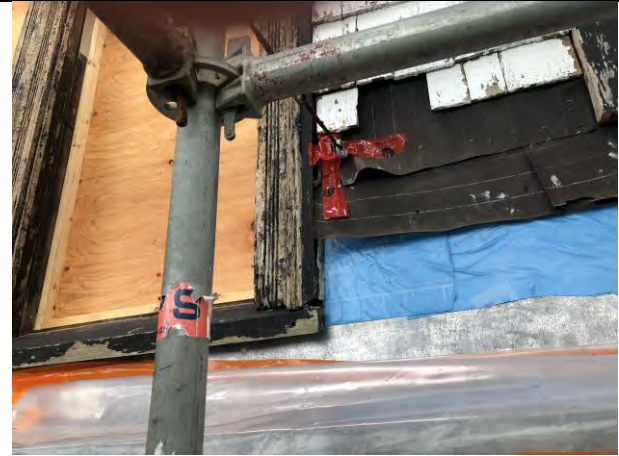
Figure 12 – Shingles on the elevation are removed and permeable membrane is being installed.
