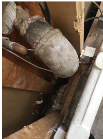
7. Existing piping & radiator
