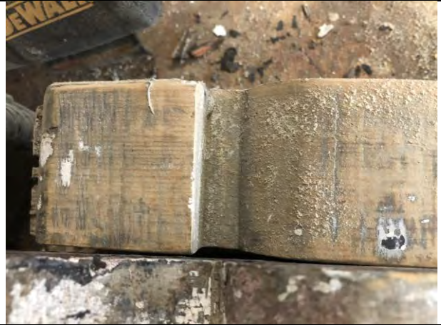
Figure 26– Detail of historic woodwork being treated in shop.
