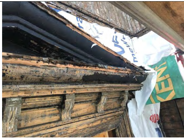
Figure 46 – Pediment to be repaired
