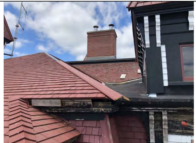
Figure 4 – in the center of the photo: area of roof to be re-shingled
