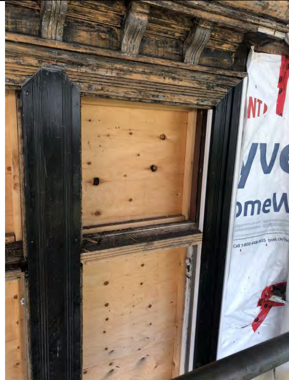
Figure 58 –Detail of transom sill. Central trim has been repaired.
