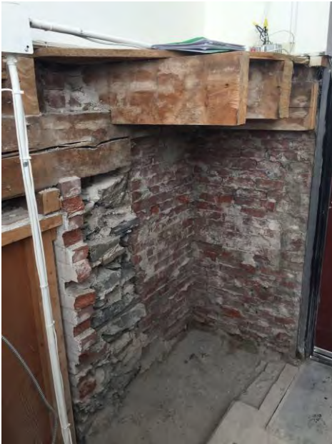
12. LHS of door, with masonry removed
