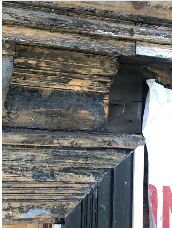
Figure 36 – Missed part. Replica of detail to be installed under pediment.
