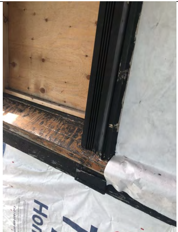
Figure 26 – Replaced window trim
