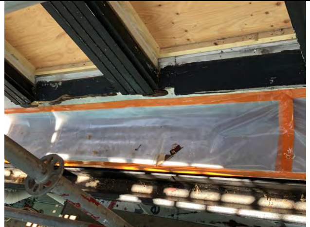
Figure 6 –area to be flashed -top of cornice
