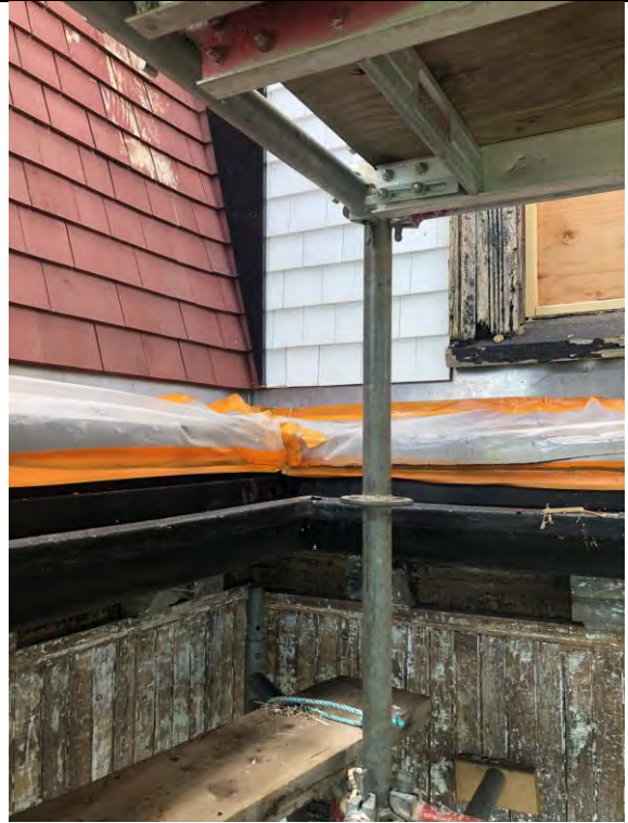
Figure 2- Roof and shingles on the 3 rd floor. Repair work in progress.
