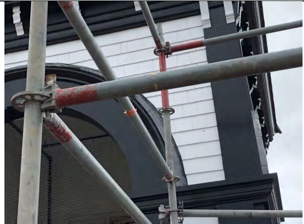
Figure 6 – Metal flashing at tower arched opening is complete.
