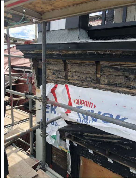
Figure 51 – Removed corbels to repair in shop.
