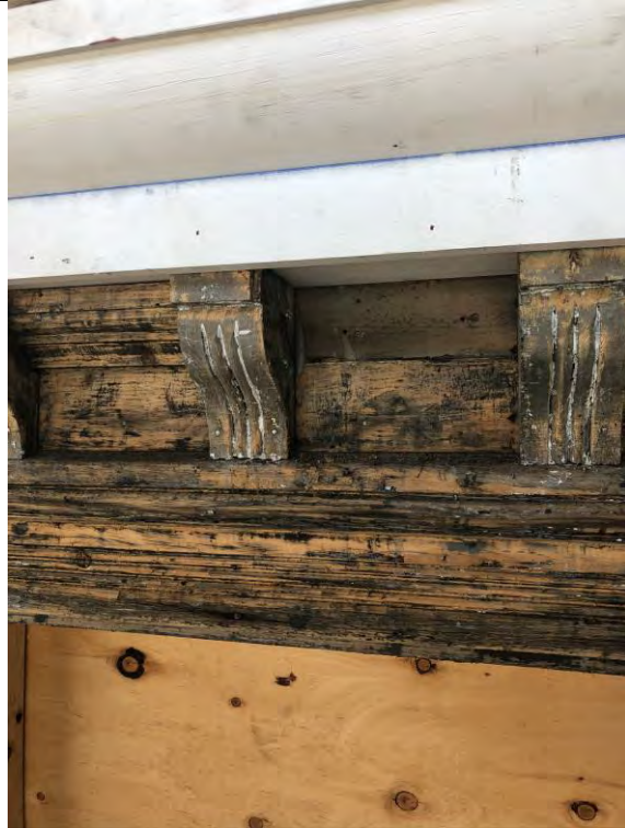
Figure 36 – Missed part. Replica of detail to be installed under pediment.
