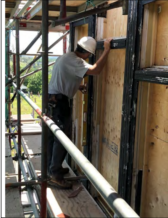
Figure 21 –Out of plumb of widows being verified.
