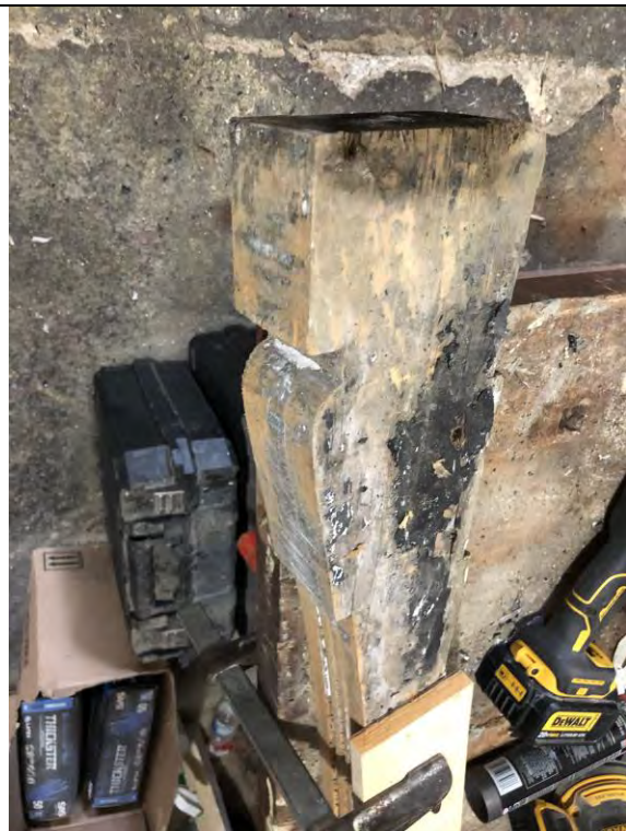
Figure 28– Detail of historic woodwork being treated in shop.
