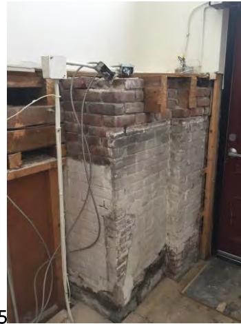
5. Masonry to be removed for new door
