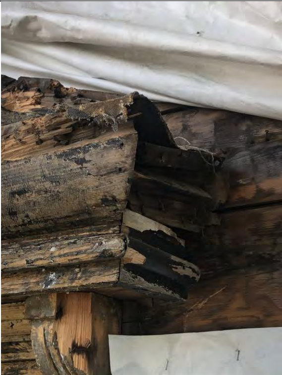
Figure 39 – Pediment. Rotten and broken wood at corner.
