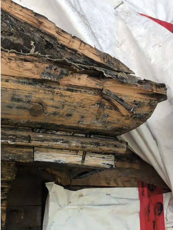
Figure 39 – Pediment. Rotten and broken wood at corner.
