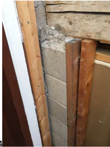
4. Projecting block wall RHS
