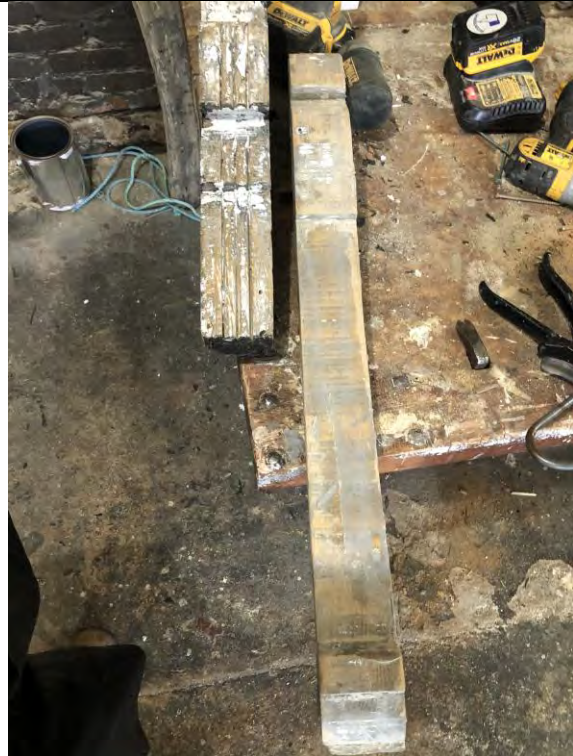
Figure 18 –Existing woodwork being repaired in shop.
