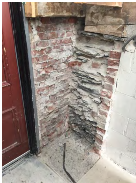
13. RHS of door, with masonry removed
