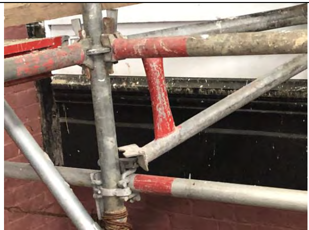
Figure 24– Detail of water table at the ground level to be replaced.
