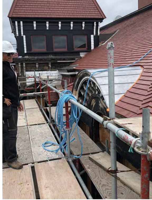
Figure 4 – Installation of lead coated copper flashing at barrel vault is completed.
