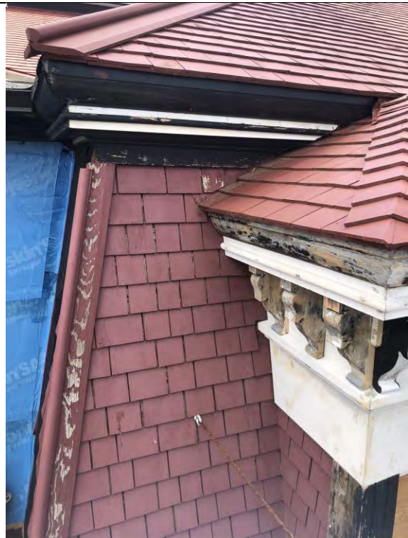
Figure 68– Detail of cladding at the side of Palladian window.
