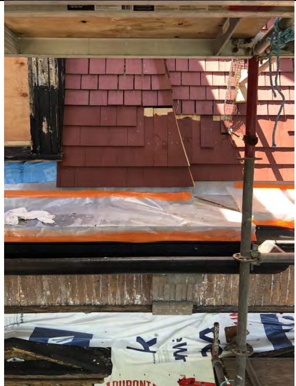
Figure 18 –Roof shingles being completed.
