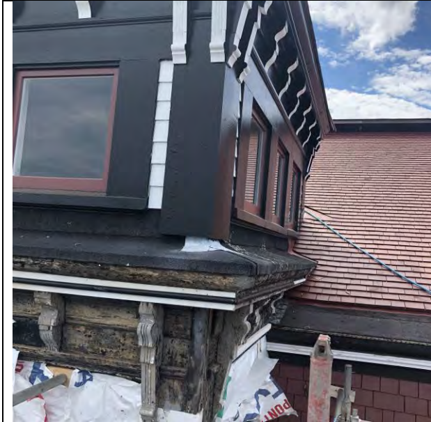
Figure 9- Asphalt on the top of the cornice on the north tower.
