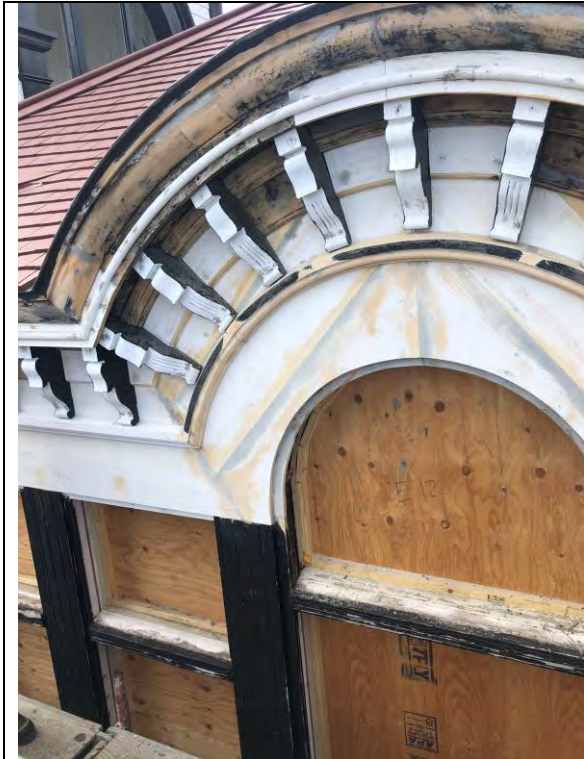
Figure 13- Wood work being repaired at the Palladian windows
