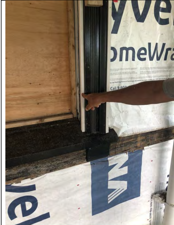
Figure 19- Wood work being repaired at the windows trims.
