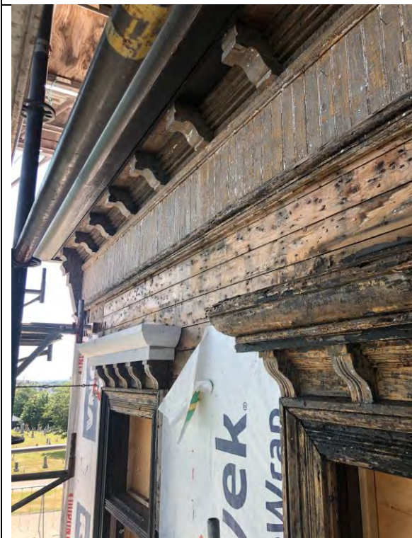
Figure 49 – Pediment repairs in progress.
