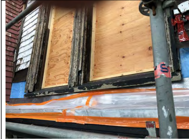
Figure 11 – Windows trims, sill and transom sills. Paint is removed and existing bare wood is exposed.
