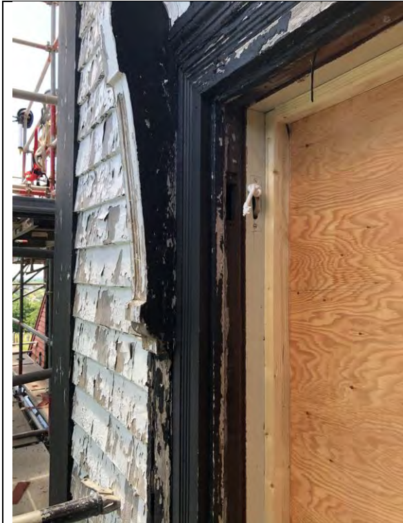
Figure 13 –Detail of trim at window during the paint removal process.
