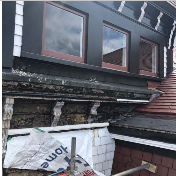
Figure 9- Asphalt on the top of the cornice on the north tower.
