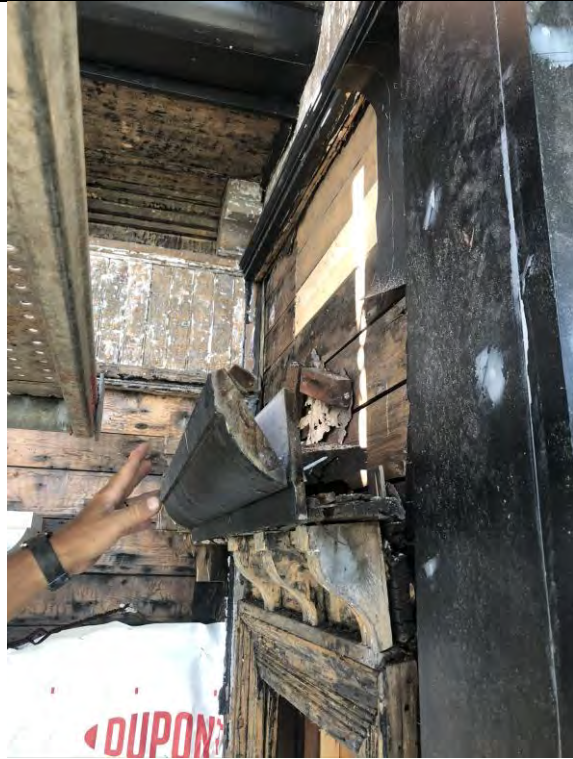
Figure 44 – Pediment in poor condition
