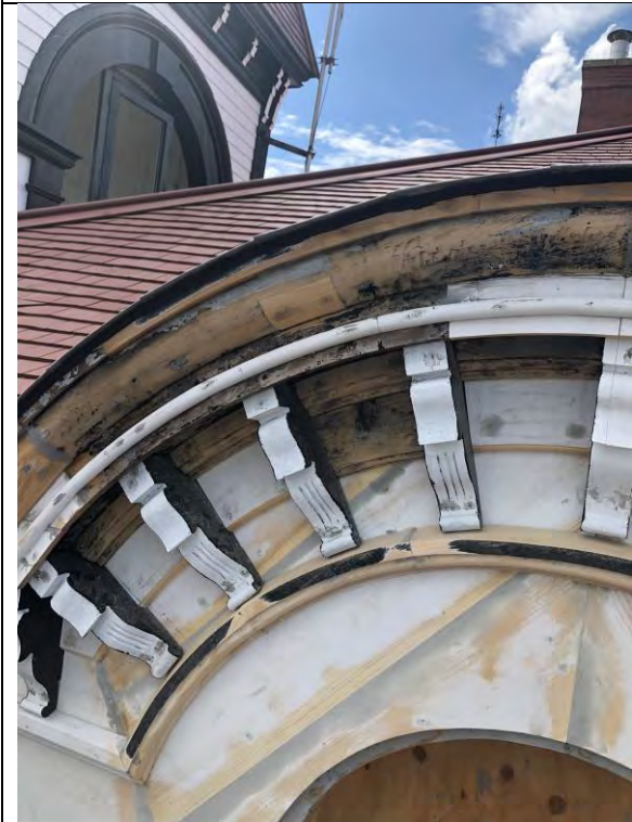
Figure 17- Wood work being repaired at the Palladian windows. Note dutchmen repairs.
