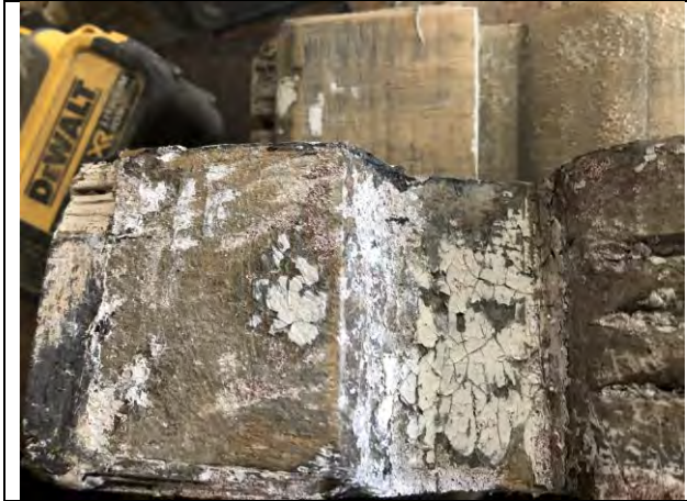
Figure 25– Detail of woodwork being treated in shop.
