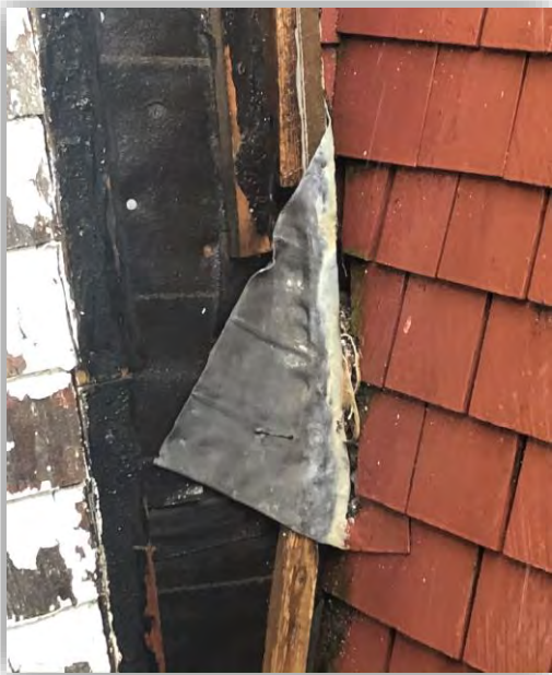
Figure 3- Existing Flashing
