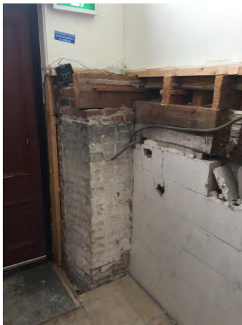
6. Masonry to be removed
