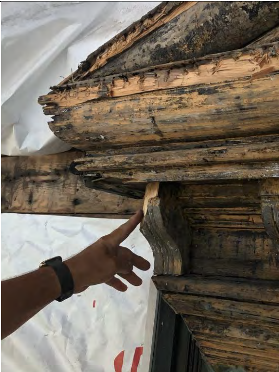
Figure 35 – Pediment to be disassembled, repaired, and reassembled. Broken wood detail.
