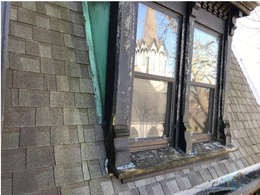
Photo 30 – Dormer with bent copper panel
