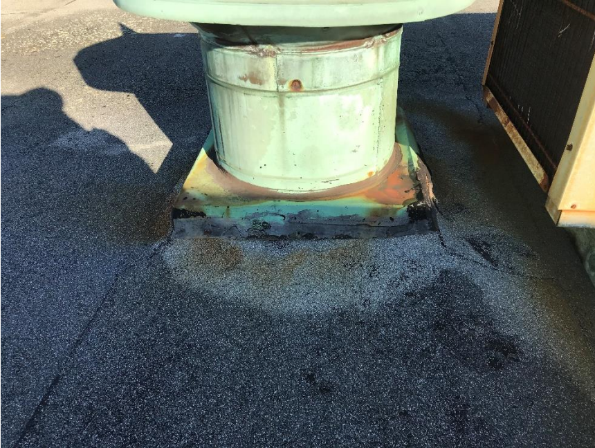
Photo 33 – Flashing around circular roof vent (1 of 2)
