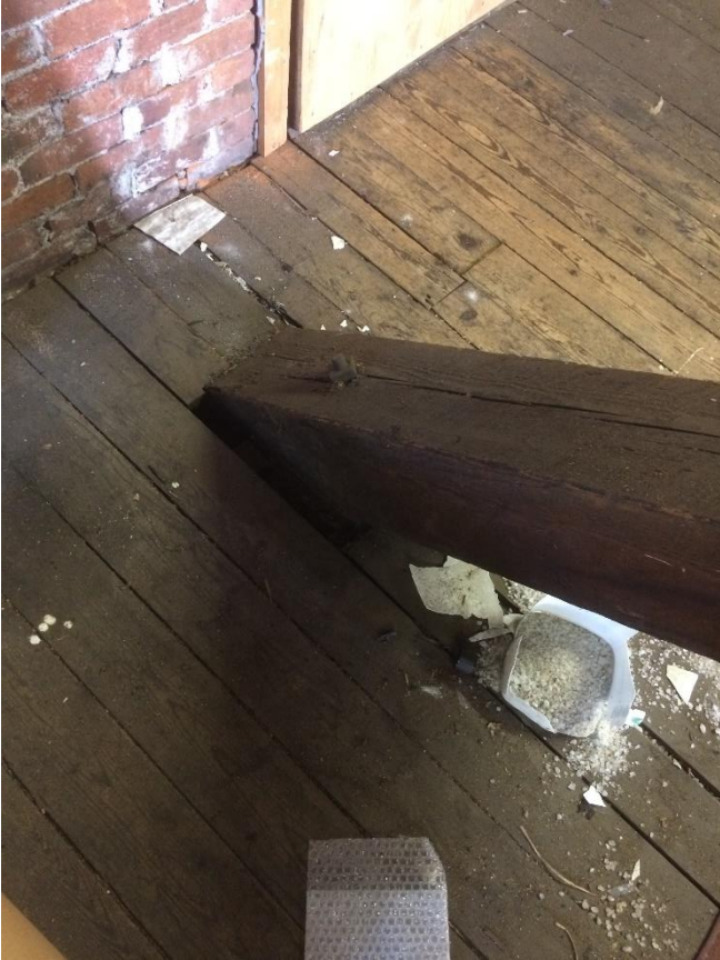
Photo 15 – Truss through-bolt connection (inclined web member to bottom chord)
