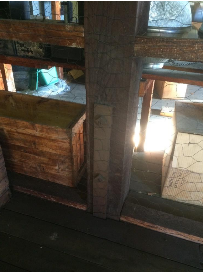
Photo 14 – Truss bracket with through-bolts
