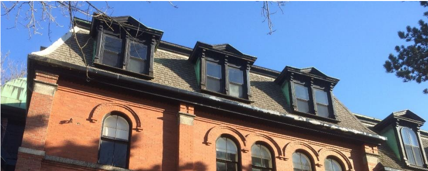
Photo 16 – Mansard-style roof on north section of building
