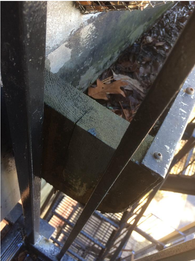
Photo 36 – Typical gutter (bent steel with wood ends)
