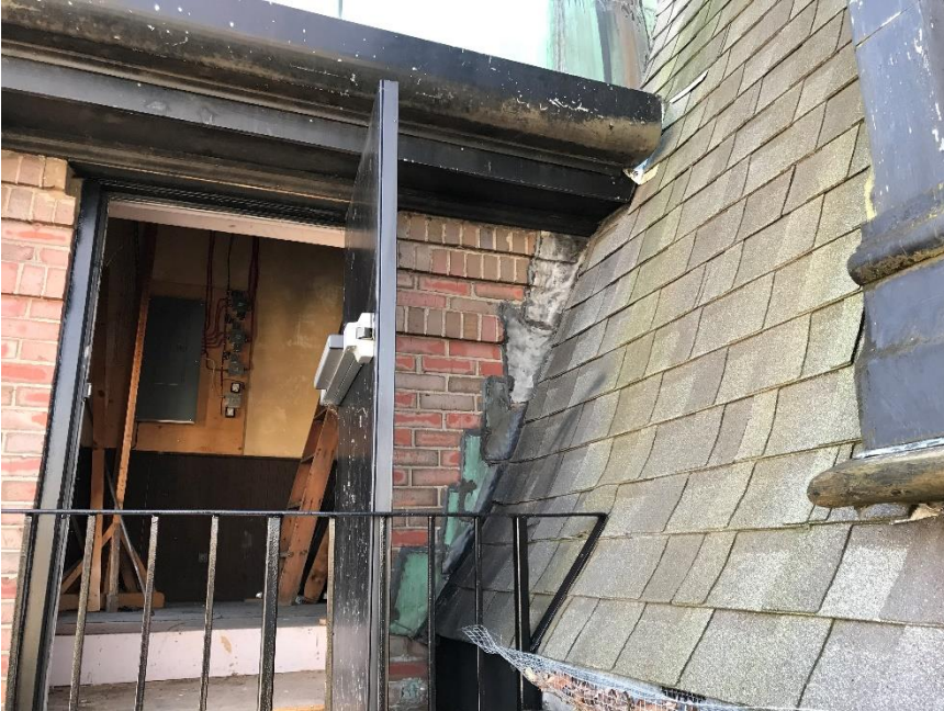
Photo 35 – Lead flashing between exterior masonry wall and Mansard-style roof
