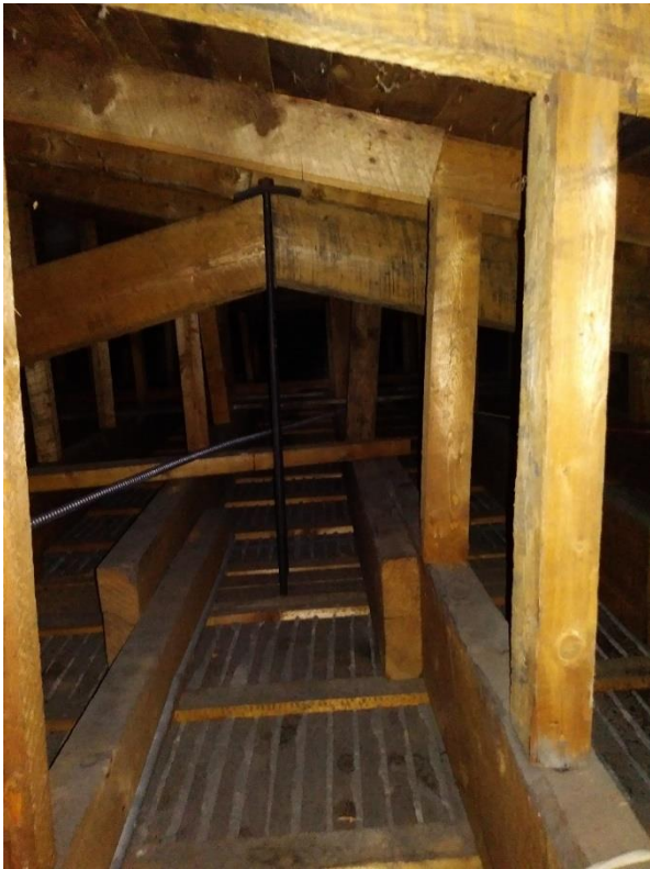
Photo 10 – Truss with double steel tension rods
