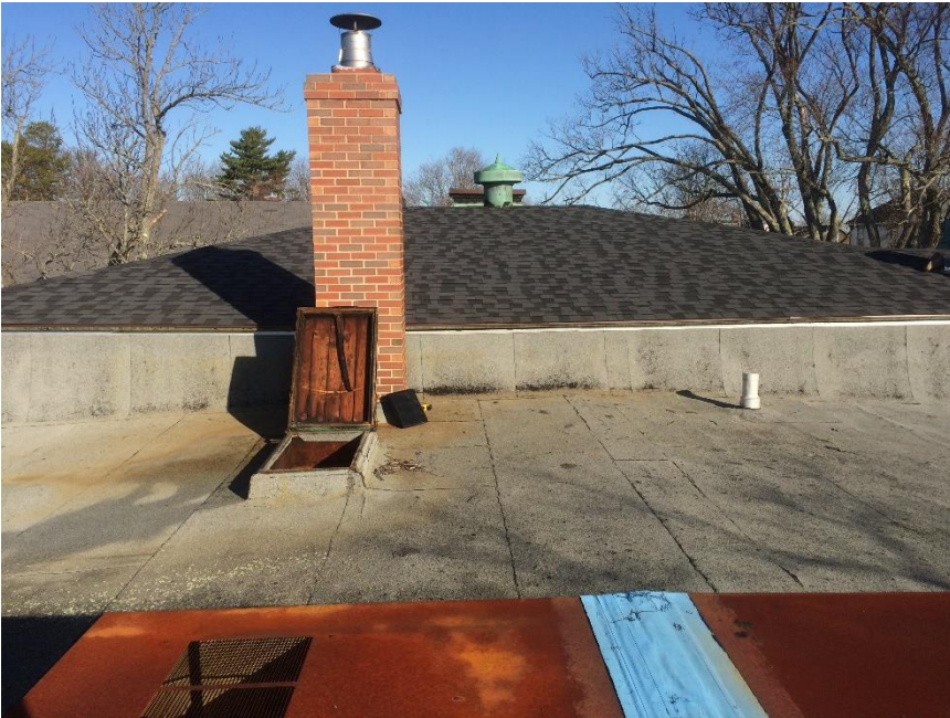
Photo 2 – Step from south roof to north roof
