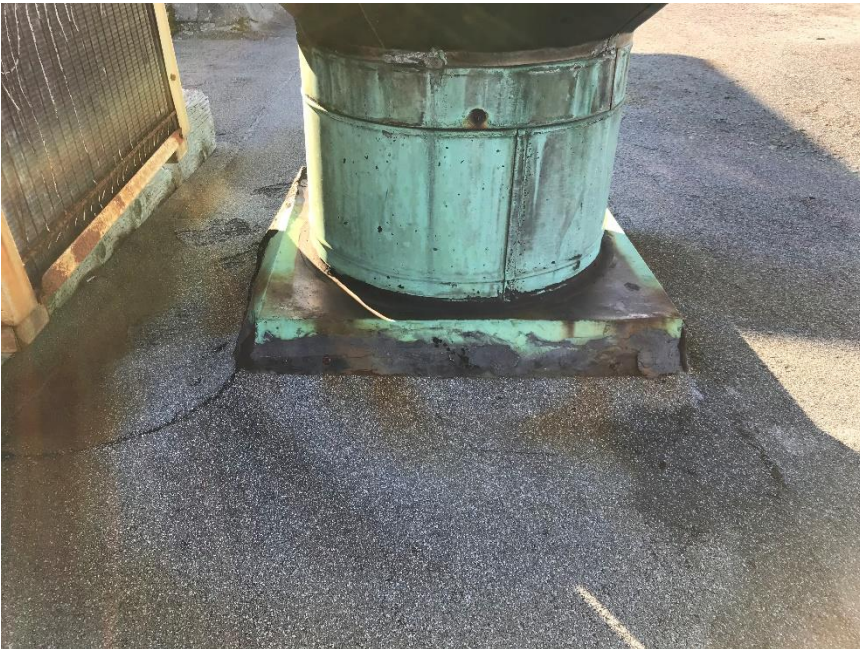
Photo 34 – Flashing around circular roof vent (2 of 2)
