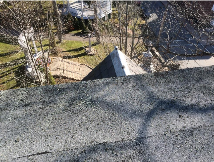
Photo 23 – Dormer with metal ridge cap
