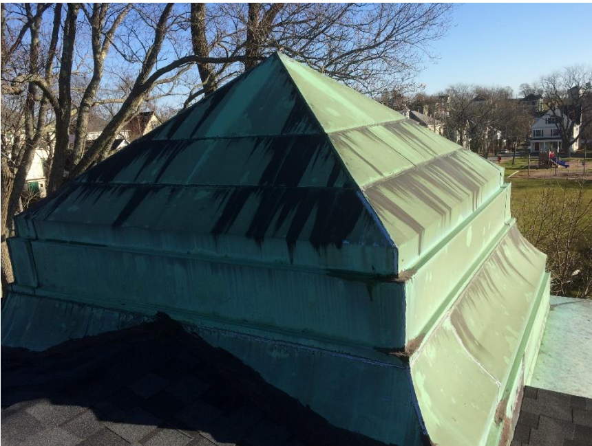
Photo 26 – Cupola with copper cover
