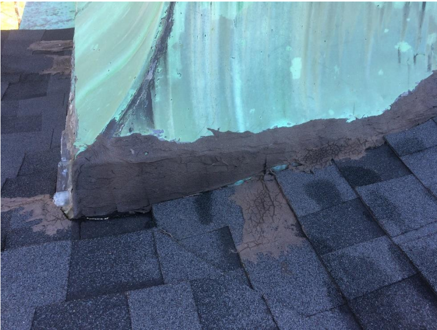
Photo 32 – Lead and tar flashing around cupola
