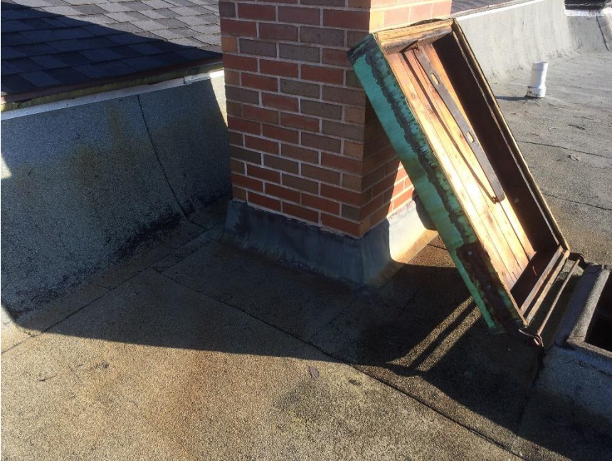
Photo 32 – Lead flashing around chimney
