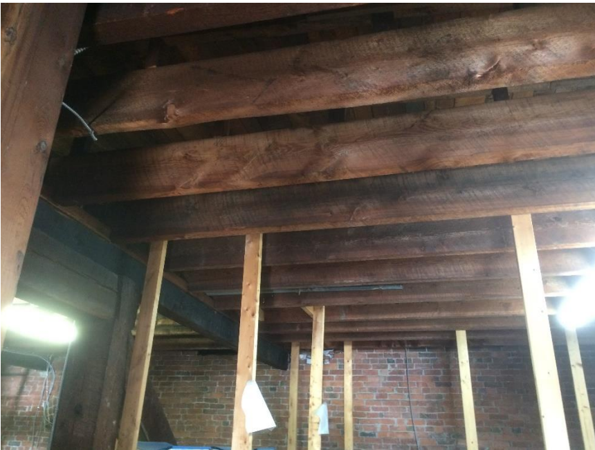
Photo 12 – Horizontal roof joists
