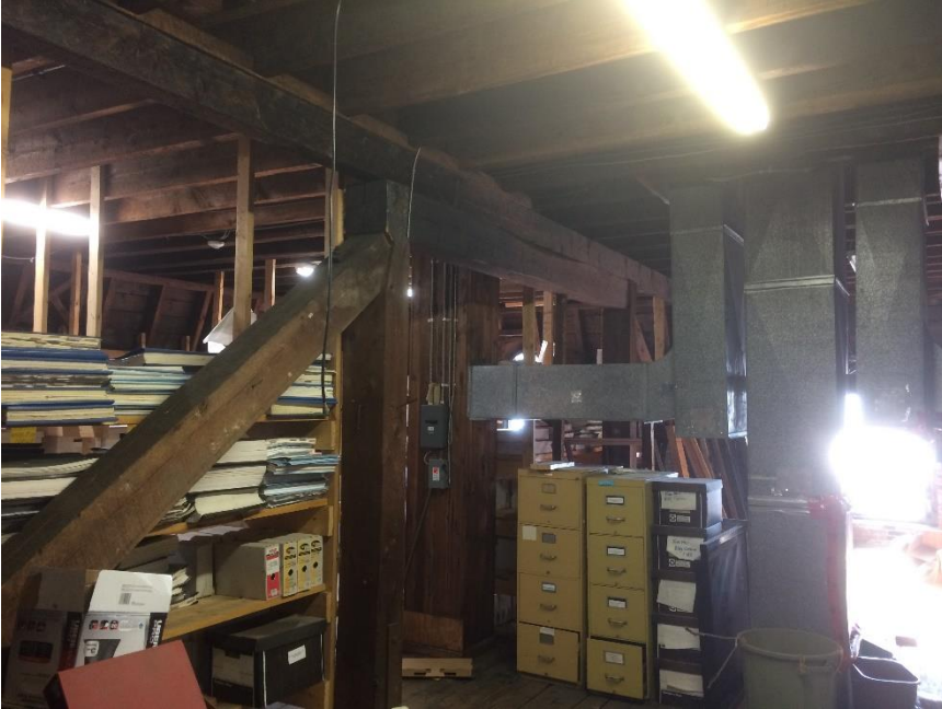
Photo 13 – Roof truss in south section of building
