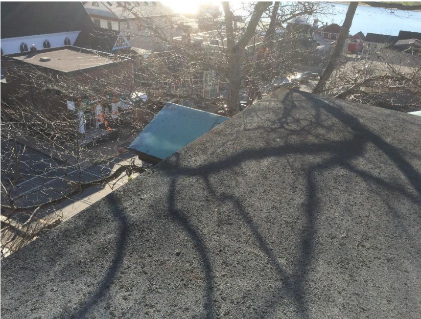
Photo 24 – Dormer with copper roof
