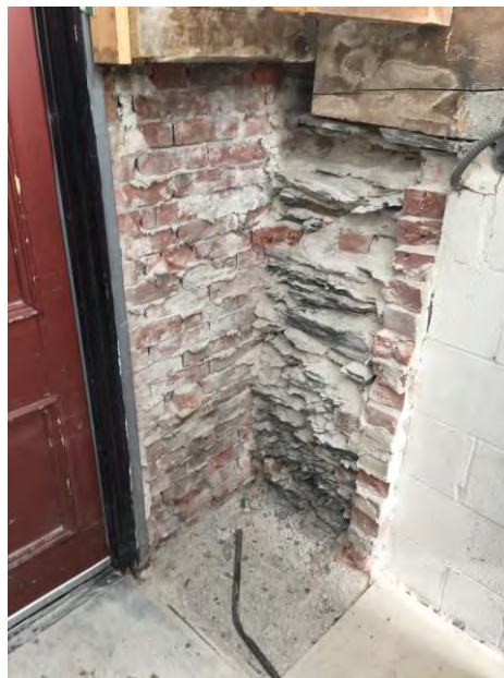
13. RHS of door, with masonry removed
