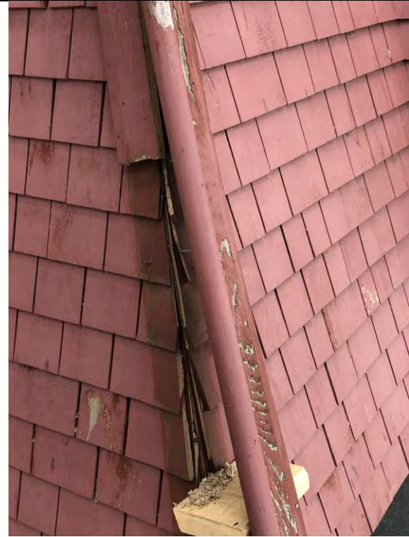
Figure 8 – Cladding on the 3 rd floor that is being repaired. Roof hip cap to be replaced.
