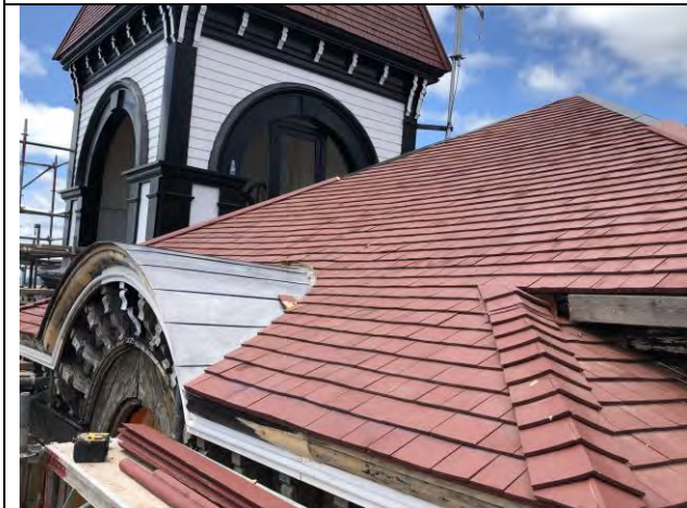
Figure 3 – Area of roof re-shingle almost complete
