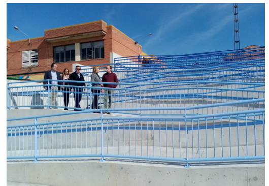
Image: Example of a concrete switchback ramp with metal handrail.
